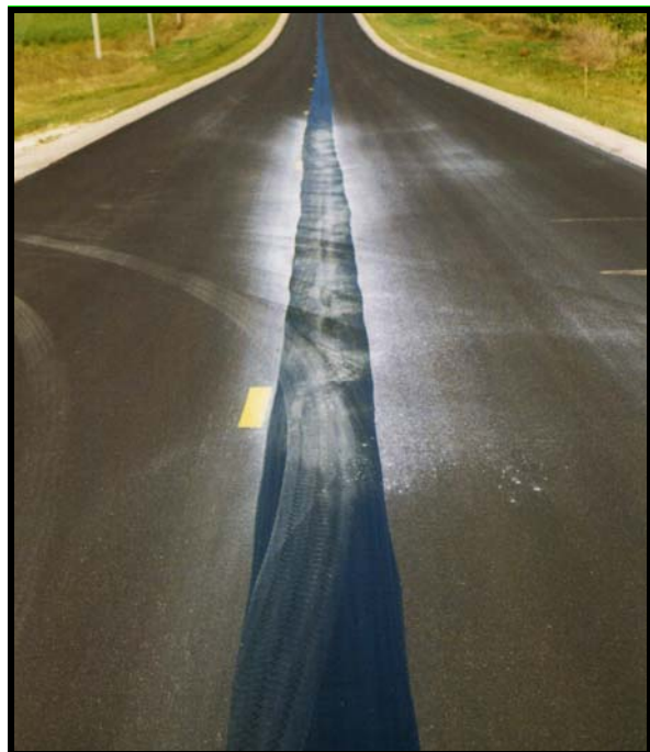
Figure 9 Application of lime dust at intersections
