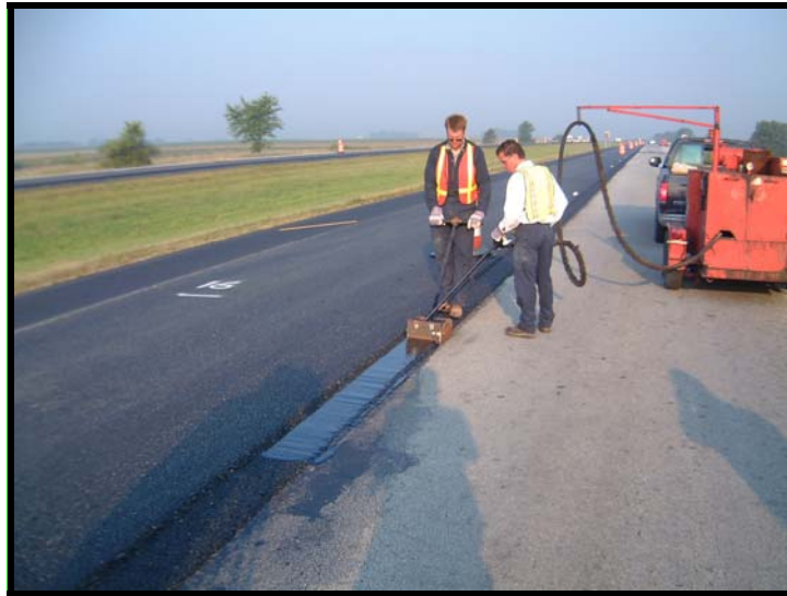
Figure 1 J-Band ® Material Placement
