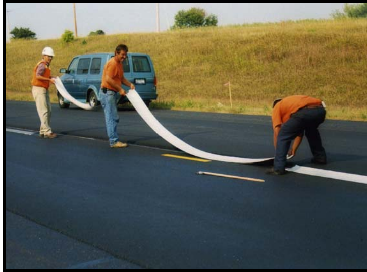
Figure 13 Placement of the QuickSeam® material
