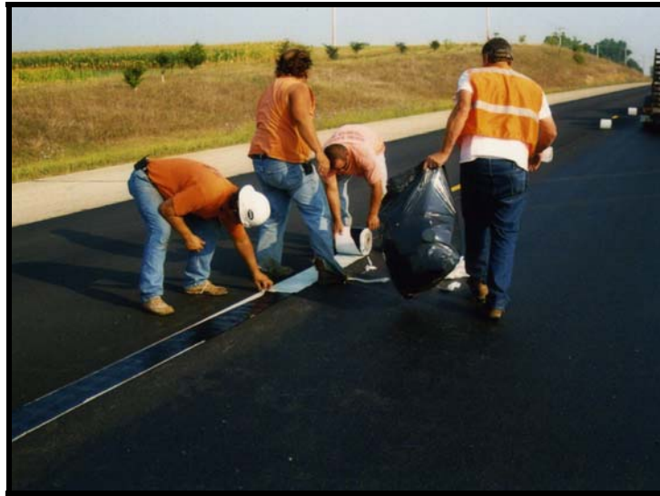
Figure 11 Removal of QuickSeam ® plastic backing
