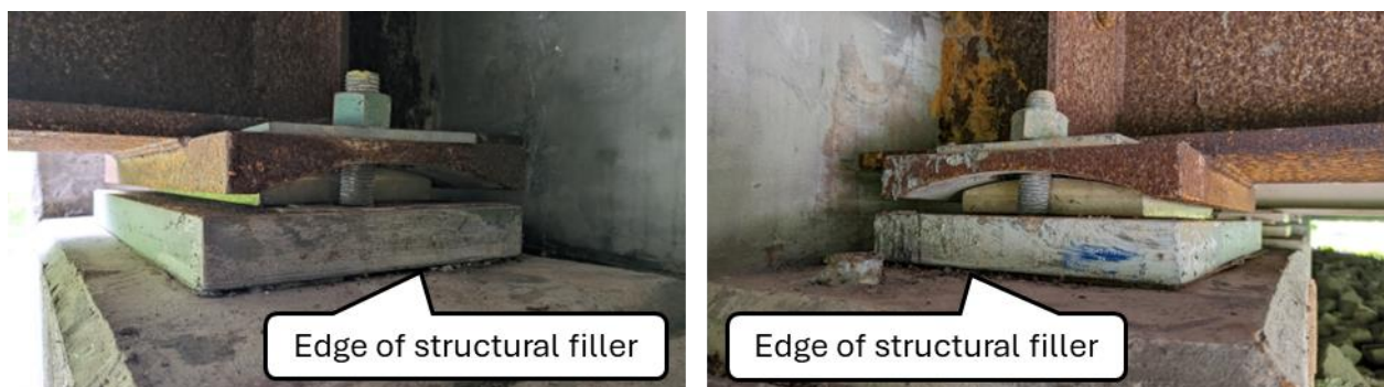
Figure 23. Photos of Bearing Preventive Maintenance Using Structural Fillers on Federal ID 24993 and Federal ID 24994 Showing Gaps Filled with Adhesive between the Top of Concrete Abutment and the Bottom of Steel Masonry Plate
