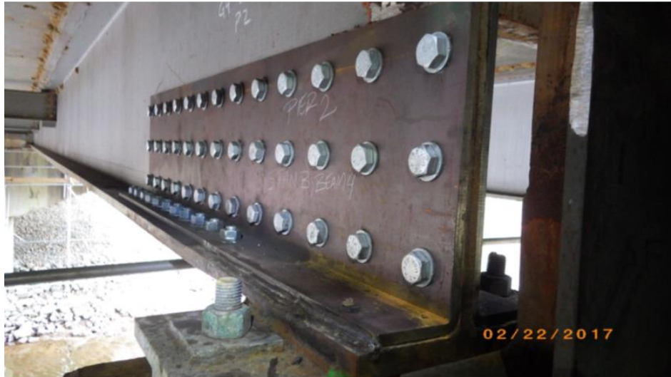
Figure 1. Steel Grouting Example with Structural Filler Used to Restore Thickness on Existing Beam with Bolted Repair Plates
