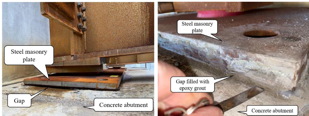
Figure 2. Gaps between Steel Masonry Plate and Concrete Abutment Seat Before (left) and After (right) Structural Fillers Were Used for Preventive Maintenance
