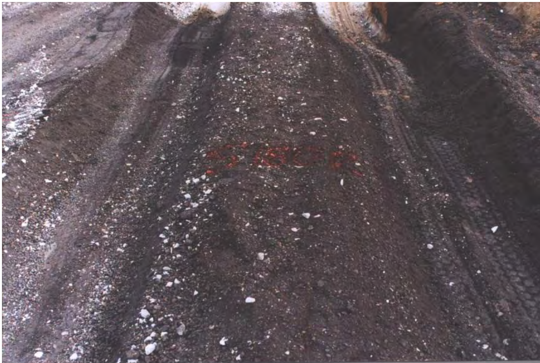
Figure 4. Test Location S180R 12" of Surface Millings after 20± Load Passes
