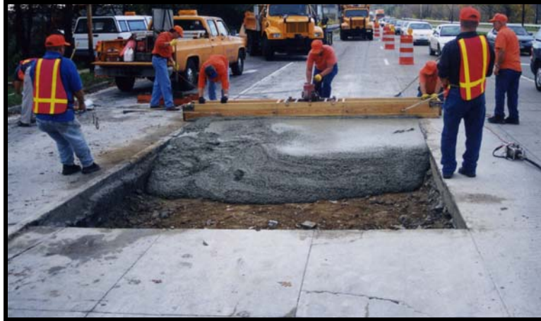
Figure 6 Full-Depth Concrete Patch Placement
