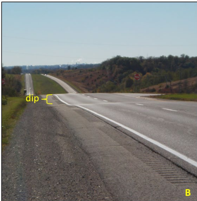
Figure 4: a- Suspected mine shaft opening on US 63 south bound near shoulder, March 2021.
