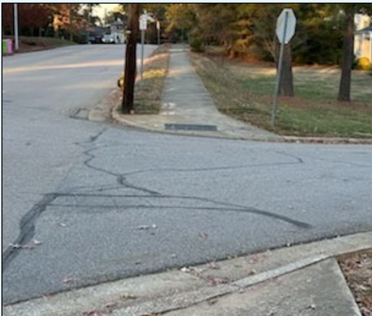
Figure 64. Photo. Illustration of an unmarked crosswalk.
