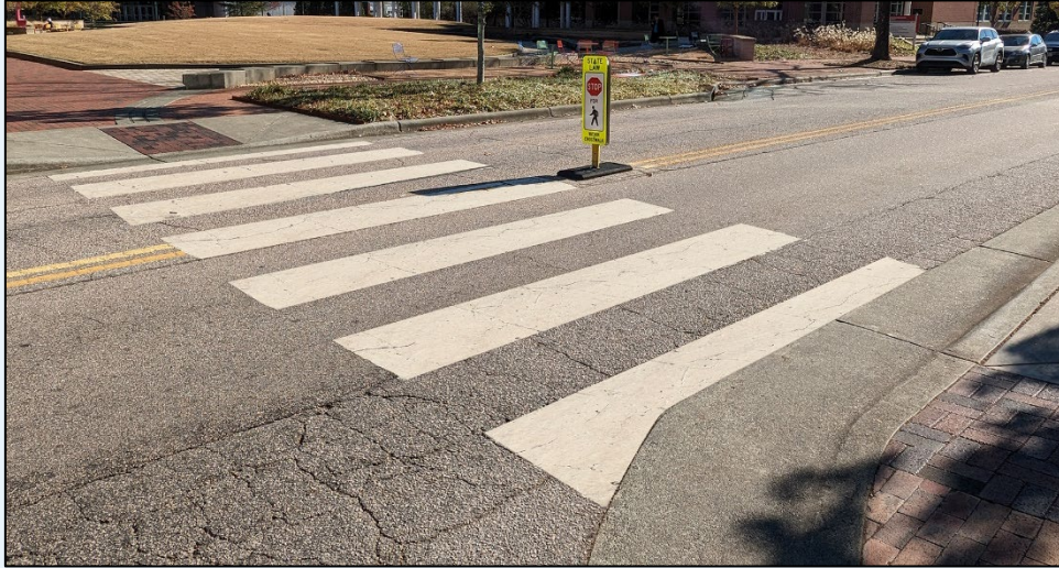
Figure 66. Photo. Illustration of a marked crosswalk with supplemental devices.
