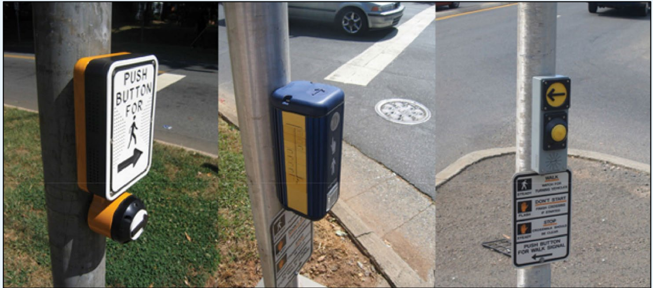
Figure 71. Graphic. Illustration of accessible pedestrian signals.
