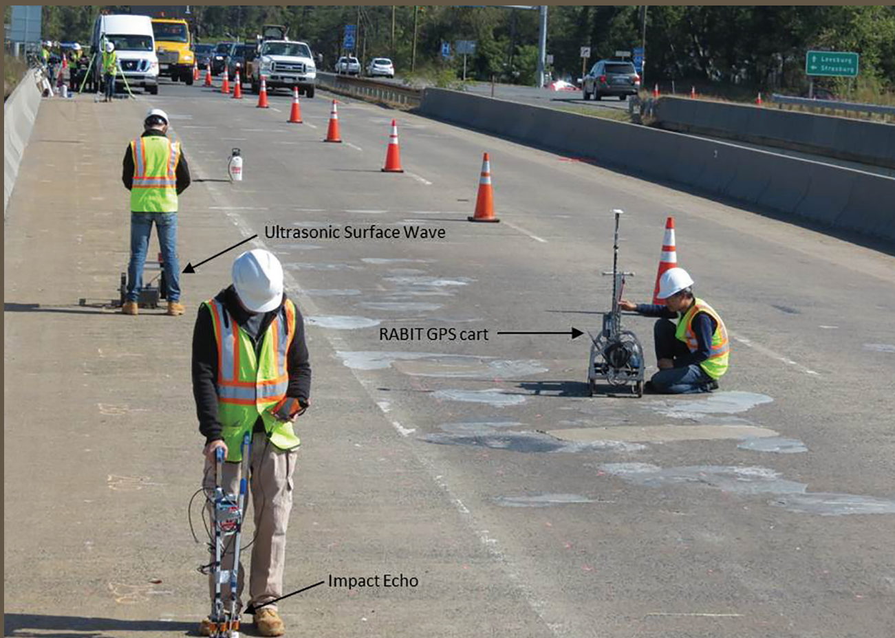
Figure 2. Data collection on the deck of the Virginia Pilot Bridge.
