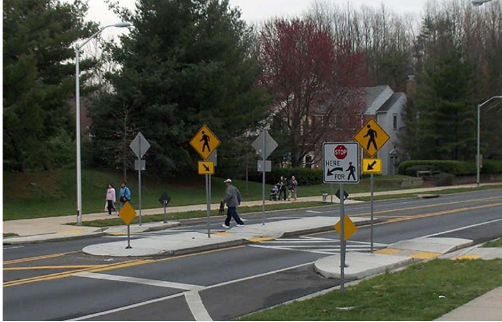
Figure 2-8. Mid-block island (Illustration: The Greenway Collaborative, Inc.)
