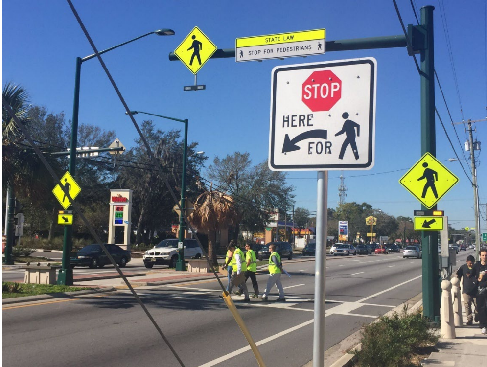
Figure 5-2. Typical RRFB Layout in Combination with Refuge Island. Source: FHP Tampa
