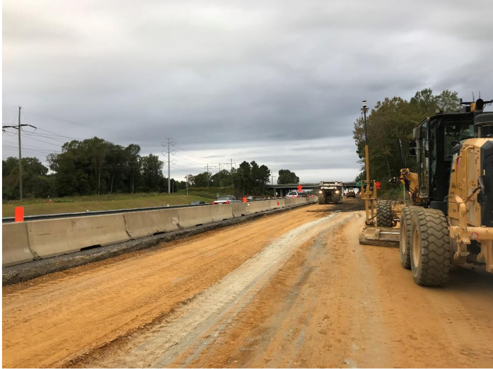
Figure A5. Subgrade Layer Placed after Excavation (October 16, 2018)
