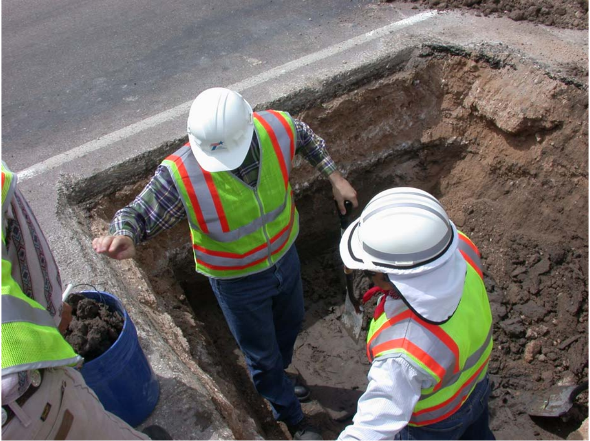
Figure B6. Collecting Samples of the Native Subgrade Material.
