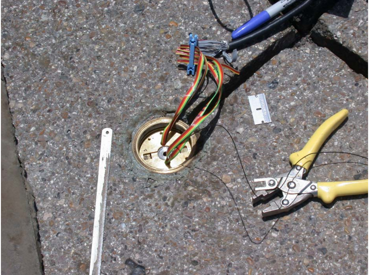
Figure B14. Setup after Installing All MDD Sensors Inside Hole.
