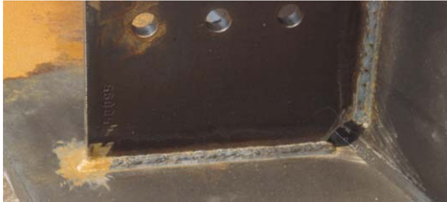
Figure 1-6: Fully Wrapped Diaphragm Stiffener
