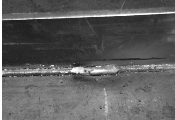
Figure 2-14: Weld Start-Stop Repair
