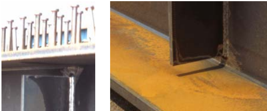
Figure 1-7: Wrapped Intermediate Stiffener Welds
