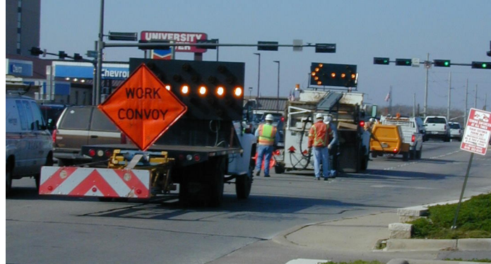
Figure 4. Crack Seal Operation in Bryan District.
