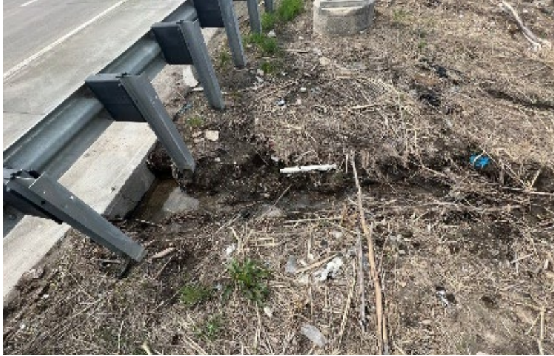
Figure 3.11: Washout Near Guardrail Near 35-46 RP 217.55
