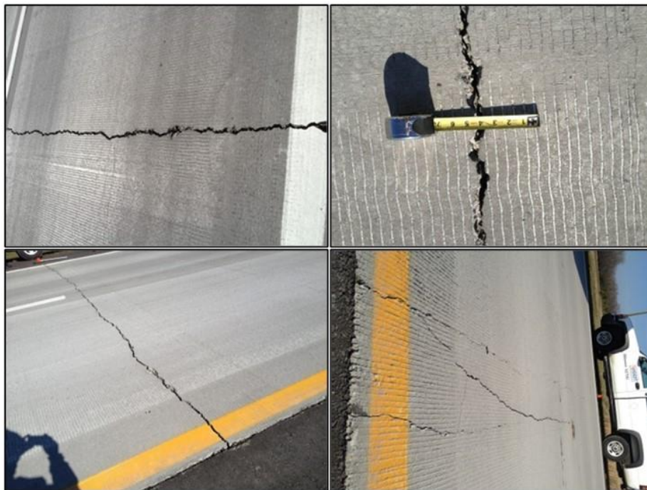
Figure 7. Bonded Concrete Surface—Wide Cracks, January 2013
