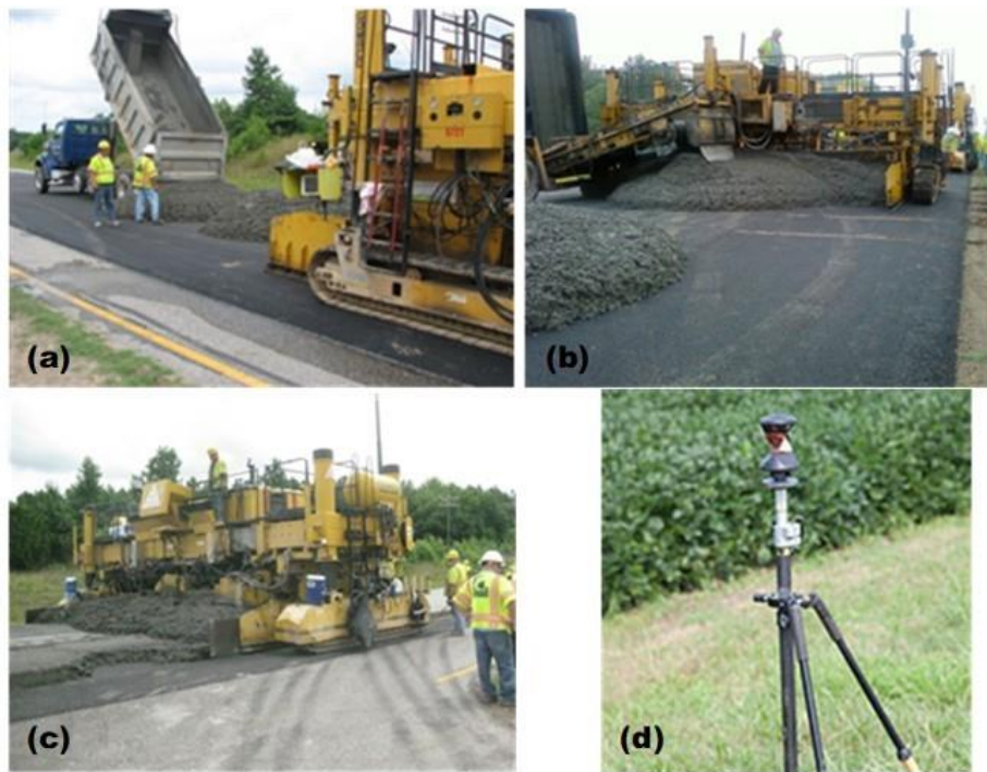
Figure 4. Paving Operation: (a) Trucks Dumping Concrete in Front of Spreader; (b) Side Discharge; (c) Two-Track Paver; (d) Global Positioning System-Enabled Laser Guidance System (Sprinkel et al., 2014)
