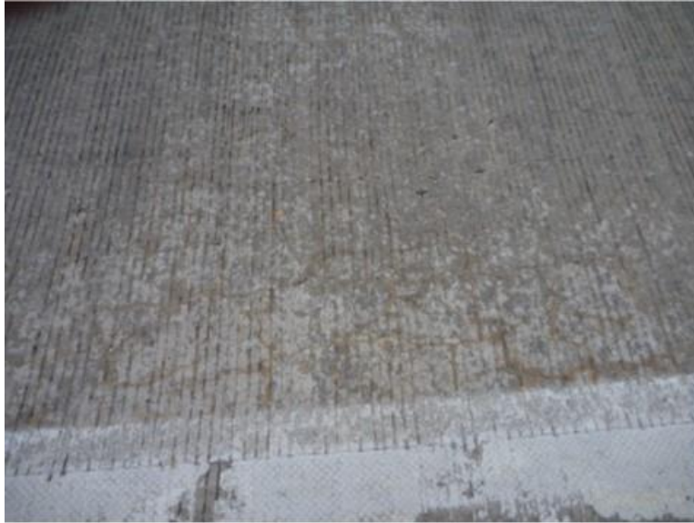
Figure 12. Map Cracks on the Patches
