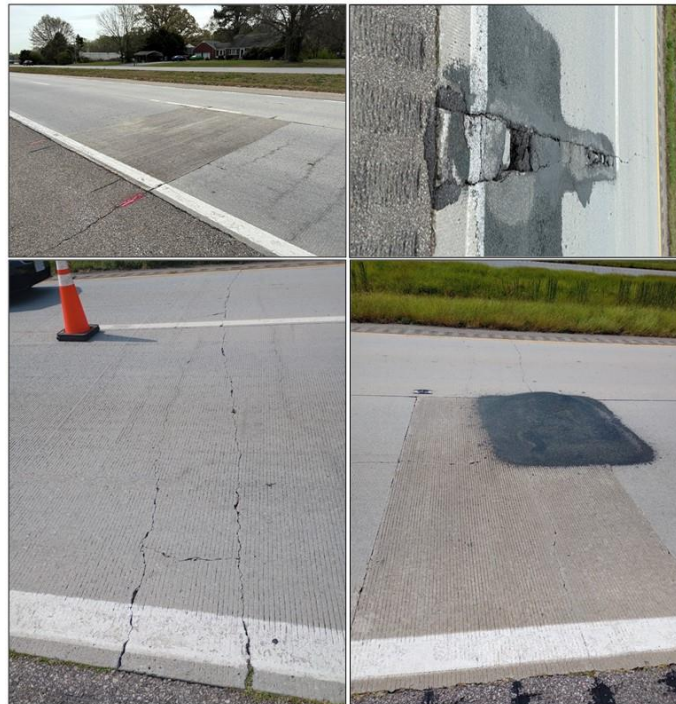
Figure 11. Surface Distresses on Bonded Section in 2025
