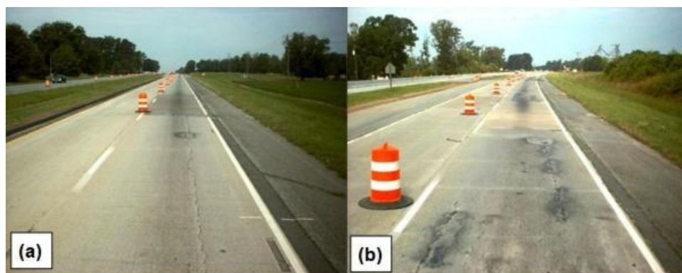
Figure 2. Distresses before Overlay, Travel (Outside) Lane: (a) Bonded and (b) Unbonded
