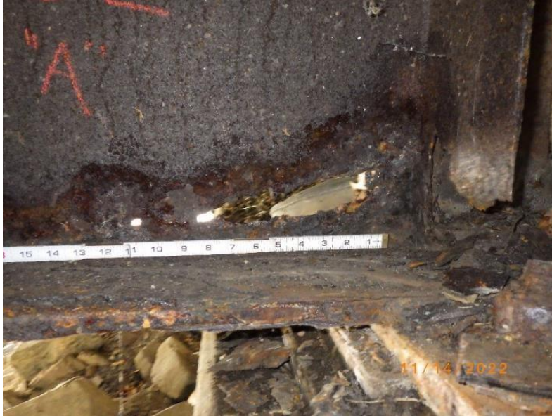
Figure 6. Example of Beam End Corrosion Damage on Bristow Road Bridge Before FRC Repairs
