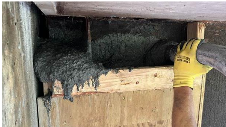
Figure 18. Photo of Bristow Road Bridge Repair Installation Showing Pumping Very High-Performance Concrete Mixture into Formwork
