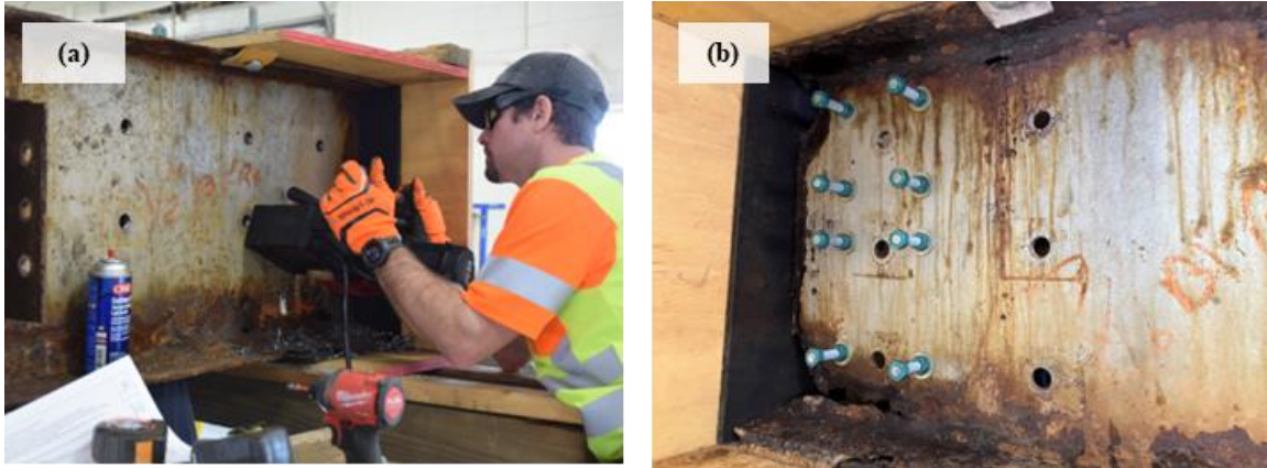
Figure 9. Installation of Threaded Rods During Mockup: (a) District Work Crew Member Using Magnetic Drill to Drill Holes; (b) Threaded Rods After Being Installed into a Beam Web
