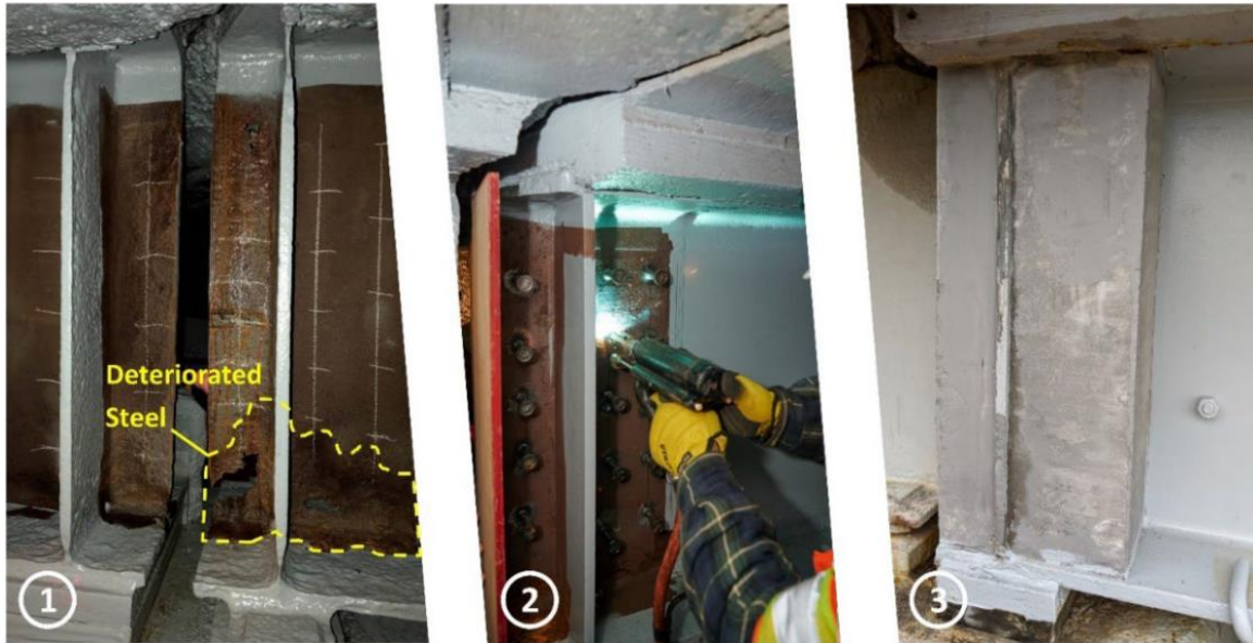
Figure 2. Photos Showing Installation of Ultra-High-Performance Concrete Beam End Repair (Haber et al., 2022)
