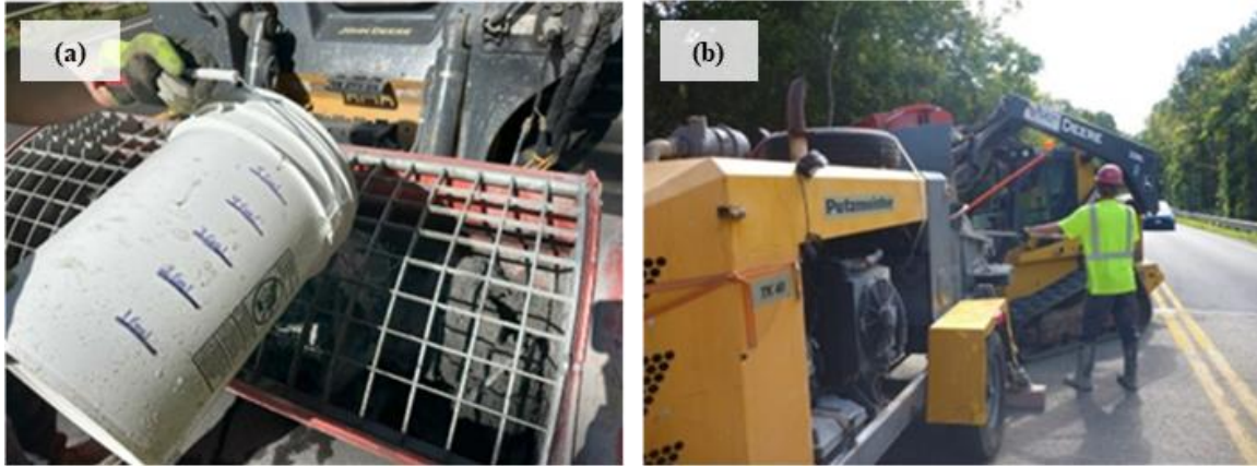
Figure 17. Photos of Bristow Road Bridge Repair Fiber Reinforced Concrete Installation: (a) High-Shear Mixer; (b) Trailer Pump
