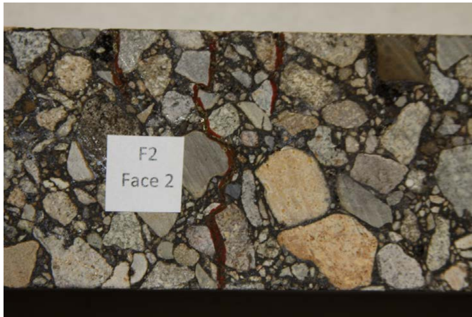
FIGURE 56 Fatigue Cracking in HMA Beam Sample SP-III-F2
