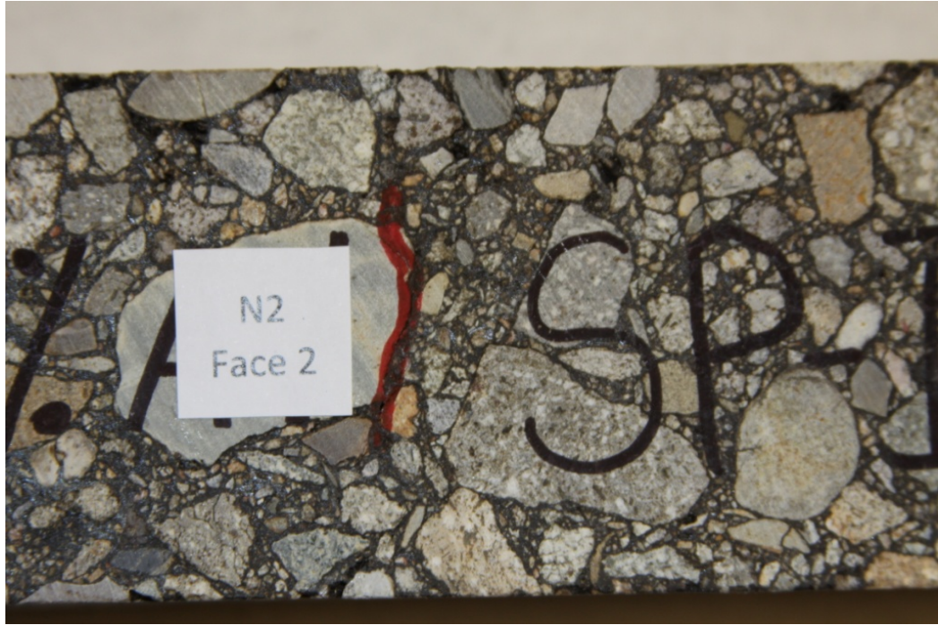
FIGURE 55 Fatigue Cracking in HMA Beam Sample SP-II-N2
