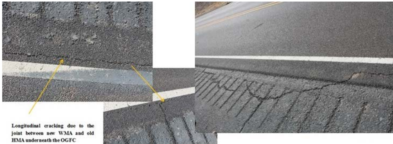
FIGURE 44 Longitudinal Cracking on the Edge of OCFC and the Existing HMA Shoulder.
