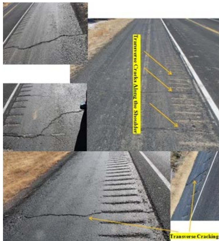
FIGURE 31 Transverse Cracking on Shoulders.
