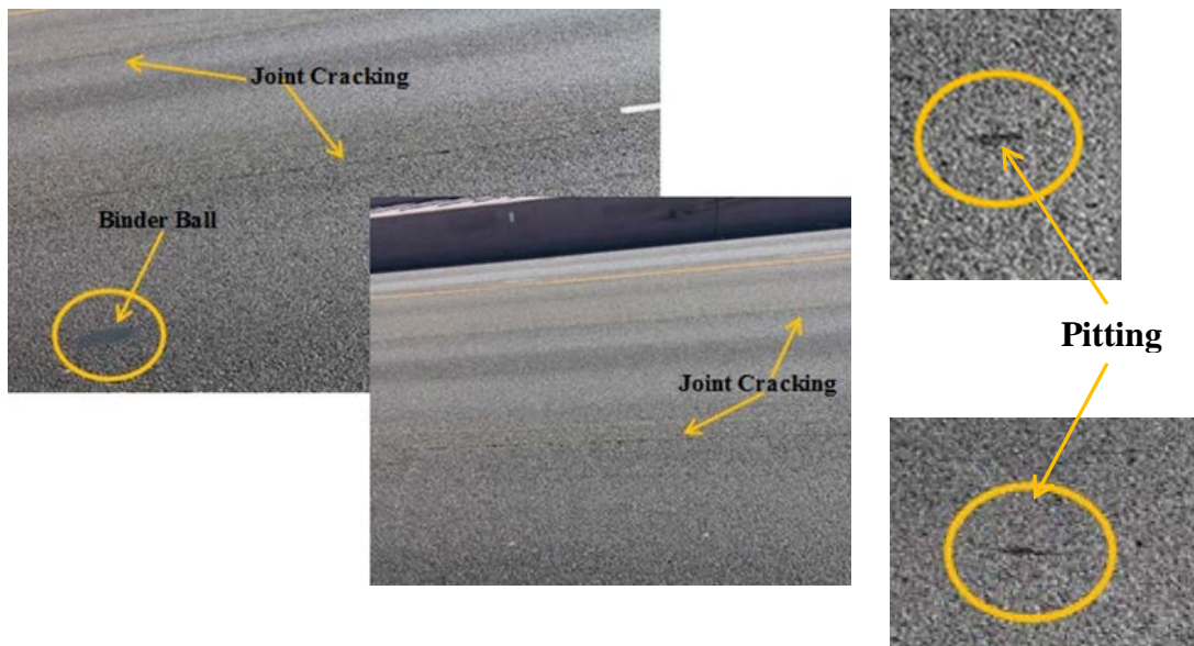
FIGURE 13 Transverse Cracking on Shoulders.
