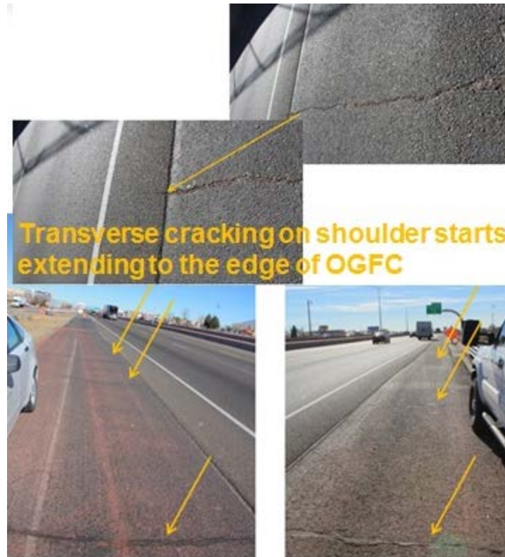
FIGURE 13 Transverse Cracking on Shoulders.
