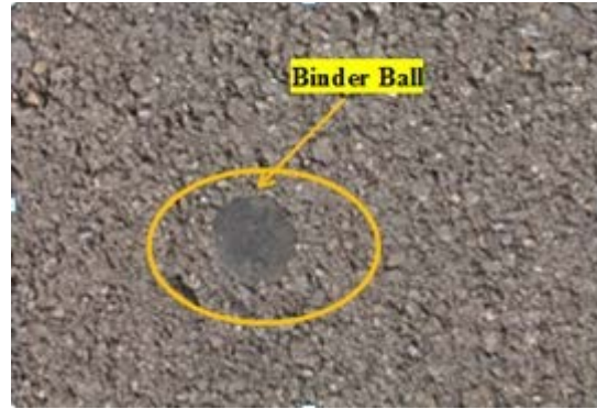
FIGURE 40 One Binder Ball Found on the WMA Shoulder.
