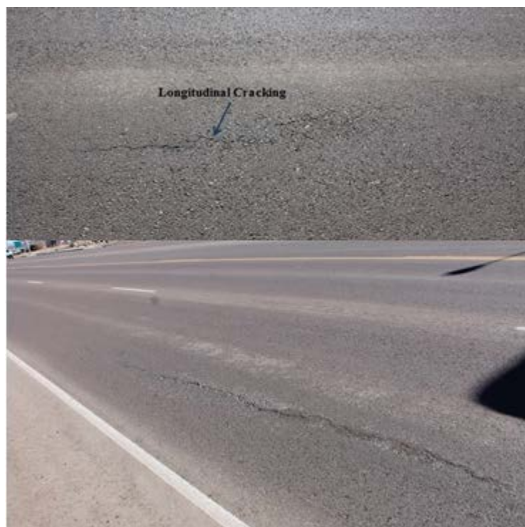
FIGURE 24 Longitudinal Cracking.
