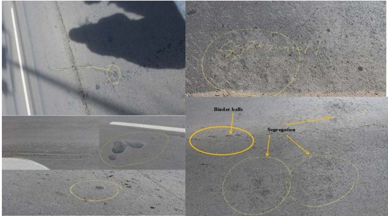
FIGURE 34 Binder Balls (Left) and Segregation (Right).
