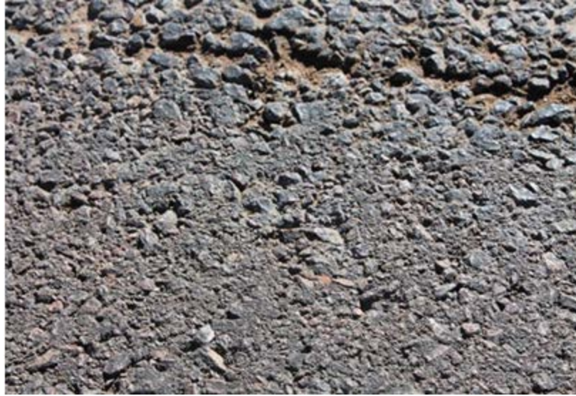
FIGURE 25 Moisture Stripping.
