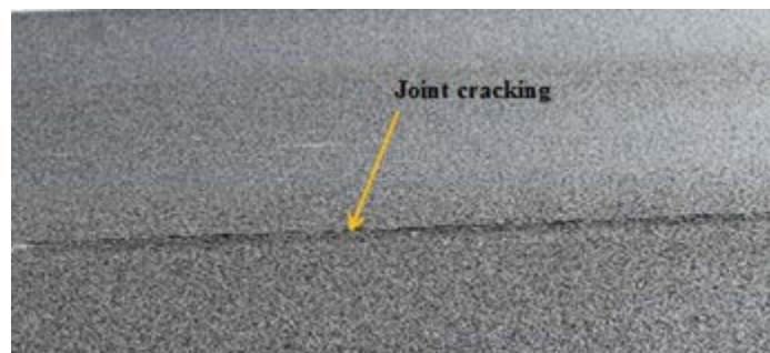
(b) Normal Joint Cracking
