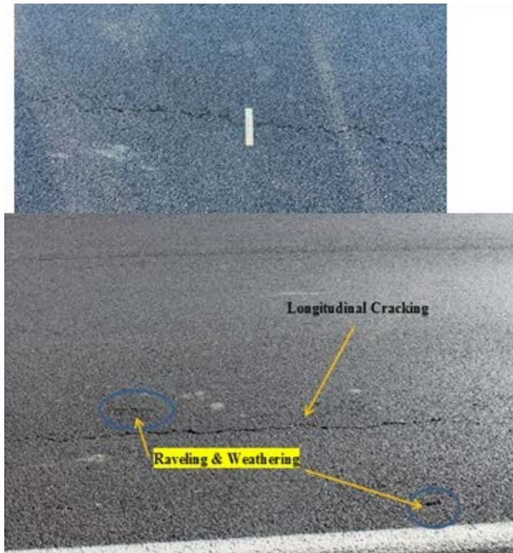
FIGURE 18 Longitudinal Cracking.
