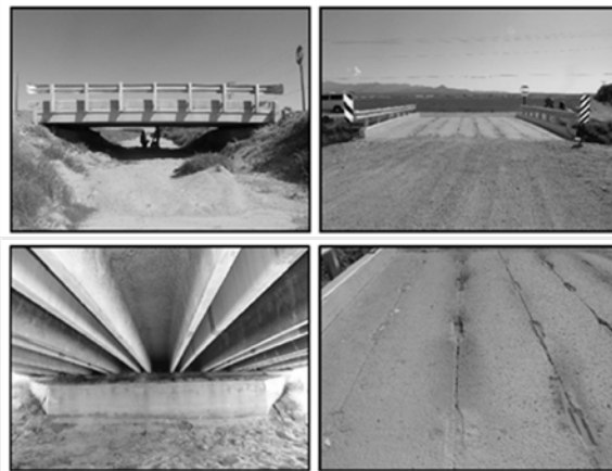
Figure 1: Prestressed Concrete Double-Tee Beam Bridge in Southern New Mexico
