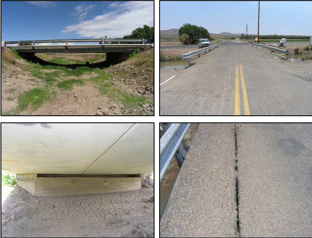
Figure 3.3. Bridge No. 7722 (prestressed concrete box girder) in NMDOT District 1.
