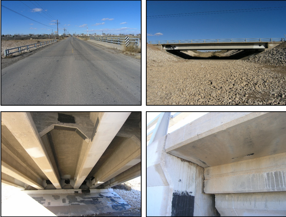
Figure 3.5. Bridge No. 8588 (prestressed concrete I-girder) in NMDOT District 2.
