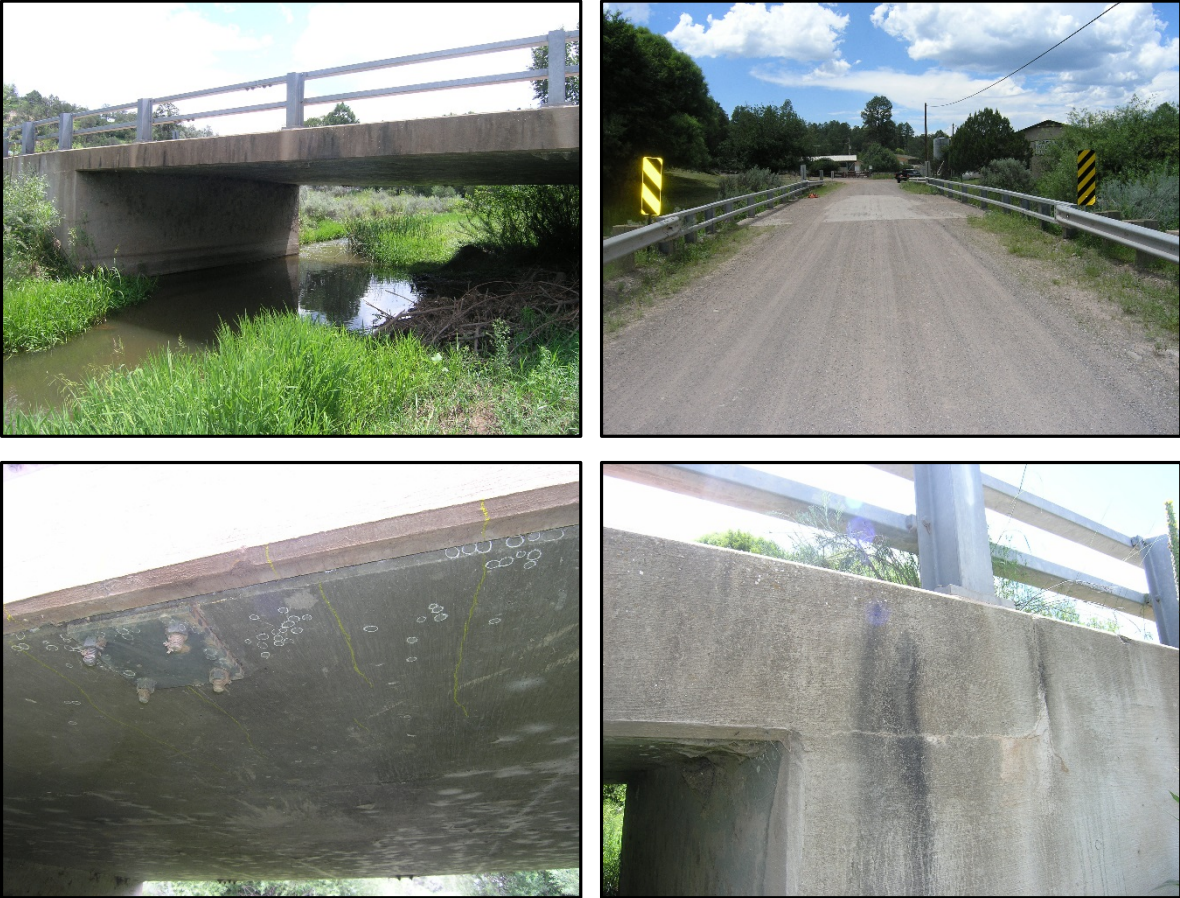
Figure 3.6. Bridge No. 8676 (reinforced concrete slab) in NMDOT District 1.
