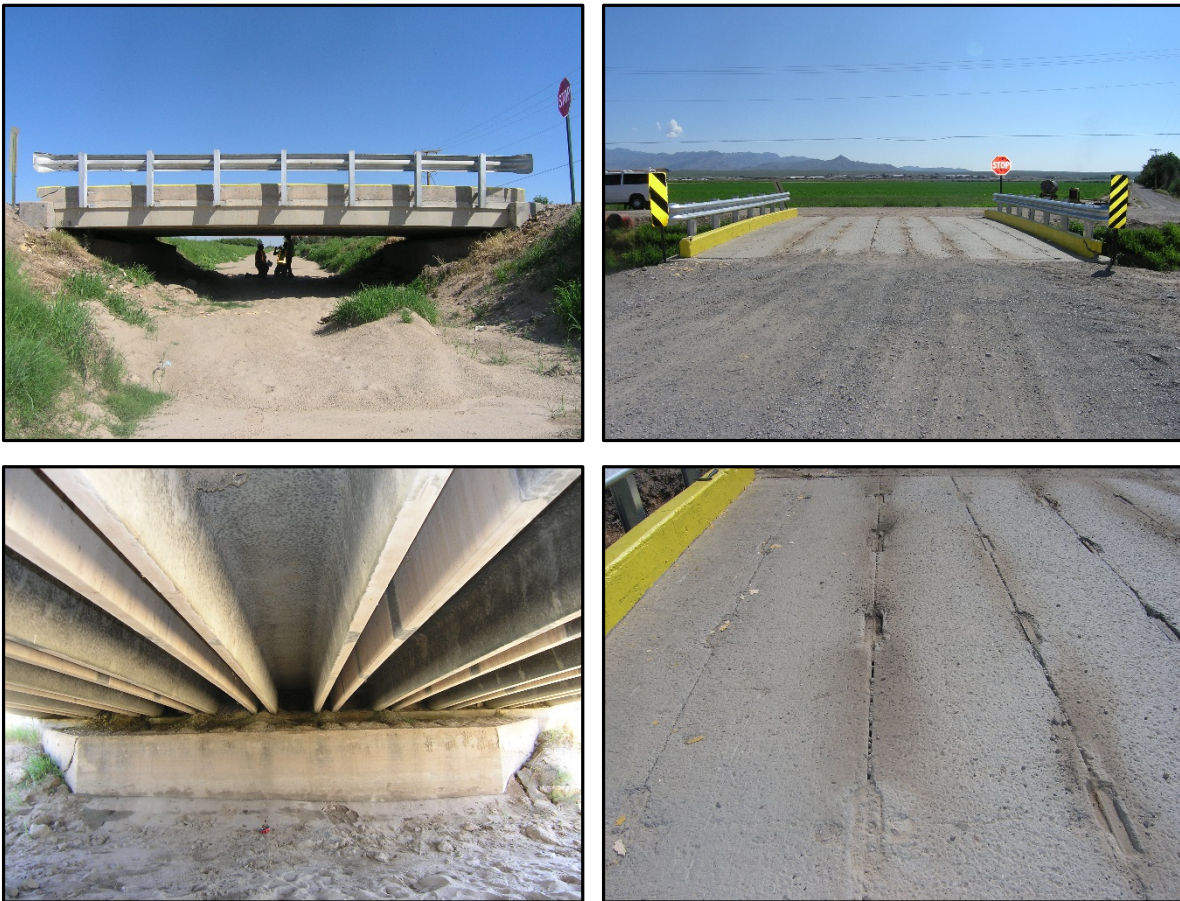
Figure 3.1. Bridge No. 7701 (prestressed concrete double T-beam) in NMDOT District 1.
