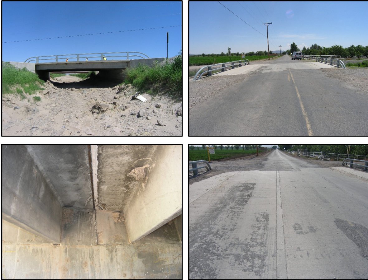
Figure 3.2. Bridge No. 8761 (prestressed concrete double T-beam) in NMDOT District 1.
