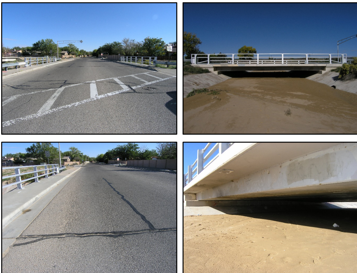
Figure 3.4. Bridge No. 8825 (prestressed concrete box girder) in NMDOT District 3.
