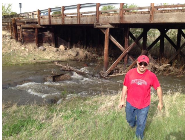
FIGURE 93 Street View of Bridge No. 1190 Showing Running Water Surrounding Intermediate Bent during the First Visit
