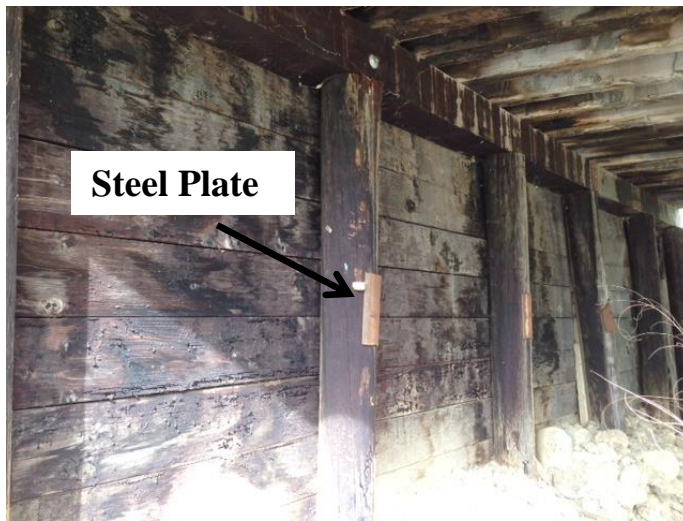
FIGURE 103 A Steel Plate Attached to Pile 10
