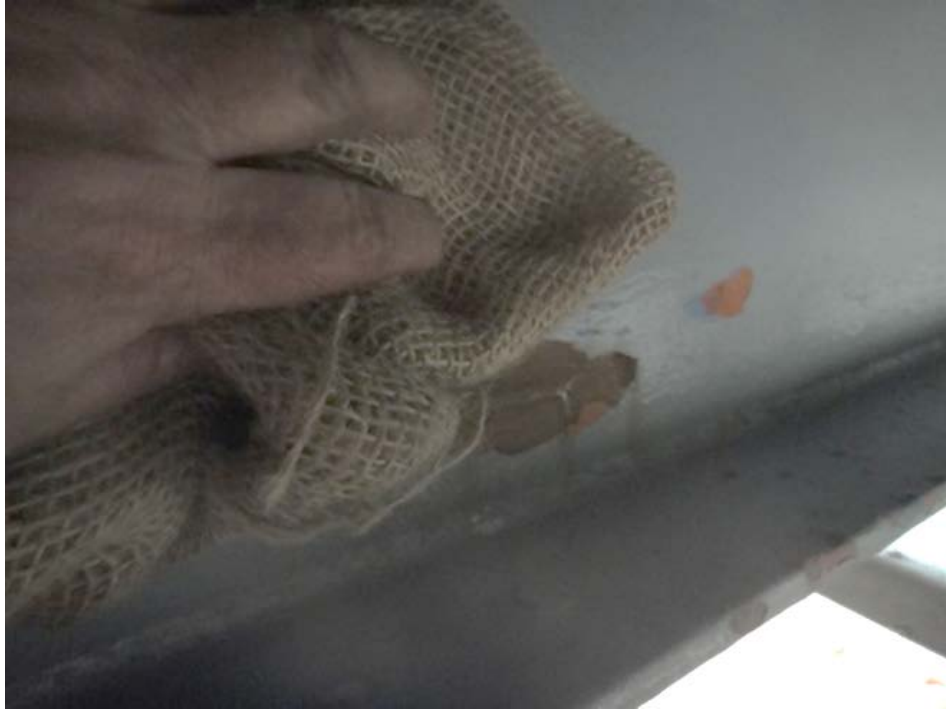
Figure 3.3 Chalking Removal with Burlap Wiping
