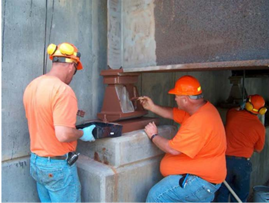
Figure 3.11 New York State DOT Technicians Brush Coating on a Bearing Note the complete patina removal by power tools on the UWS girder end in preparation for zone painting.
