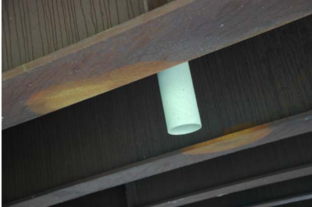
Figure 1.9 Inhibited Patina Formation on a UWS Girder Bridge
