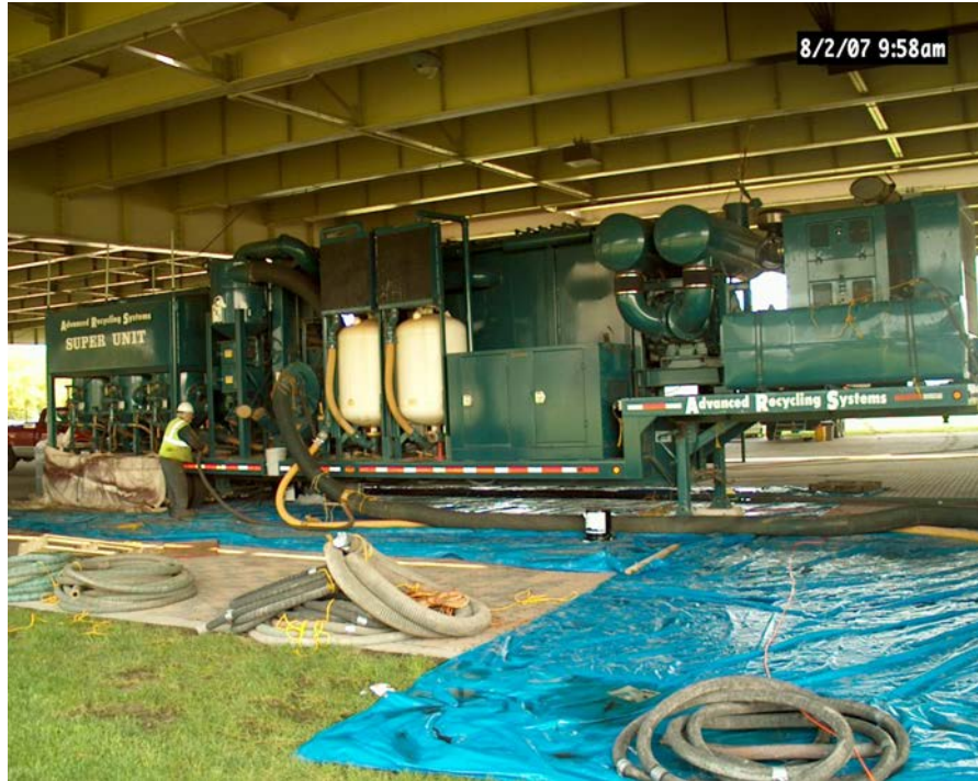
Figure 3.17 Recycling Unit on Blast Cleaning Operation
