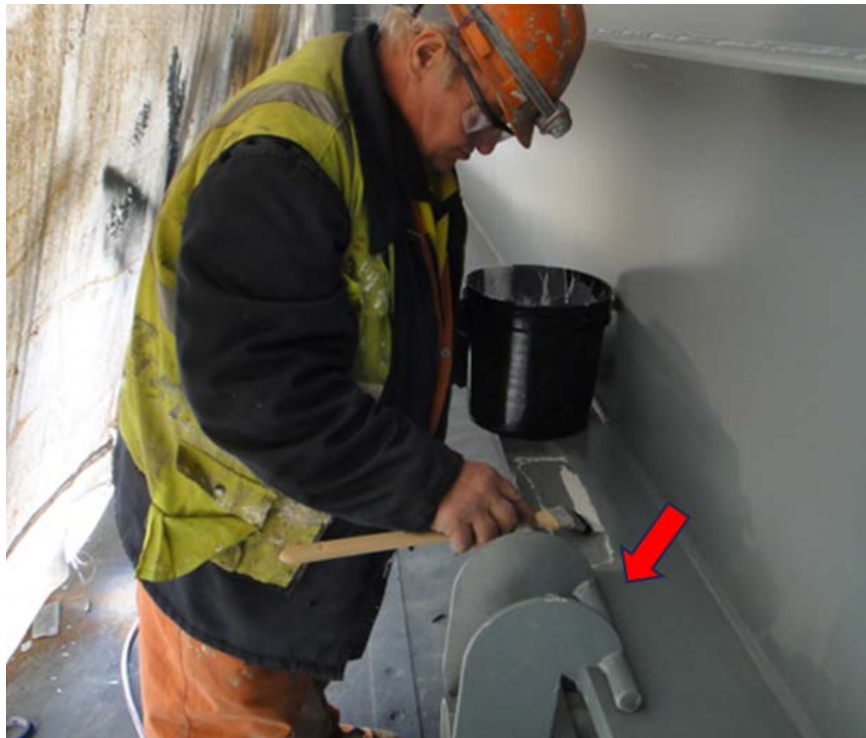
Figure 4.16 Painter Brushing a Spot Repair
