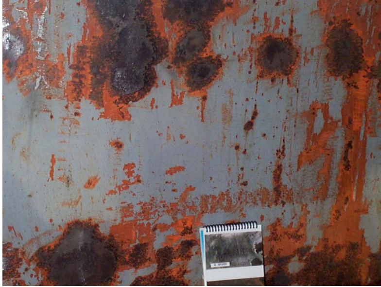
Figure 3.5 Surface Prepared to the SSPC SP-3 Standard
