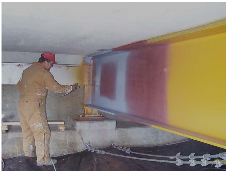
Figure 4.12 Test Patch Used as Site Standard on Overcoating Project
