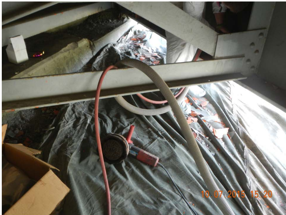
Figure 4.4 Ground Tarp Used to Collect Hazardous Waste
