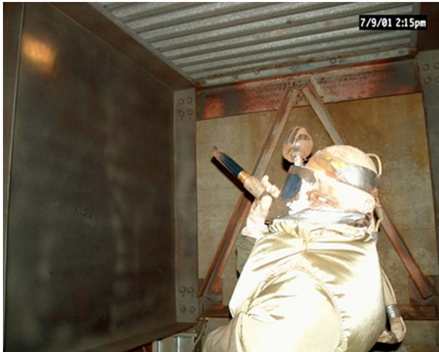
Figure 3.12 Blast Cleaning of a Girder End Prior to Zone Painting
