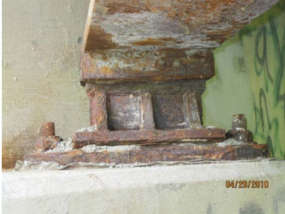
Figure 2.13 Patina Failure on UWS Beam End and Bearing
