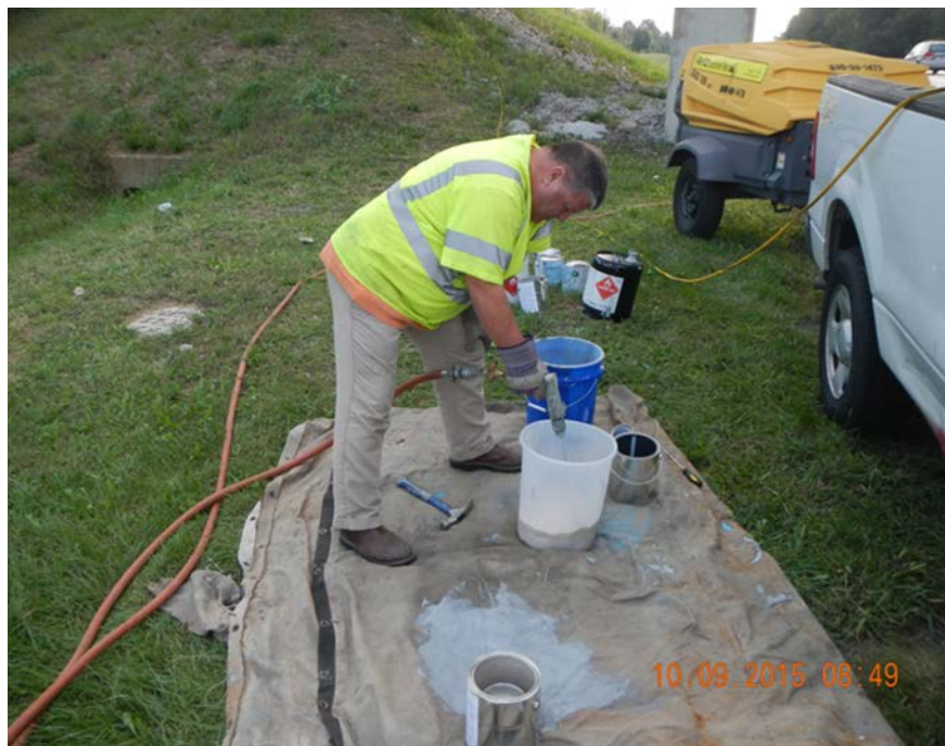
Figure 4.10 Onsite Mixing of a Multi-Component Coating Prior to Application.
