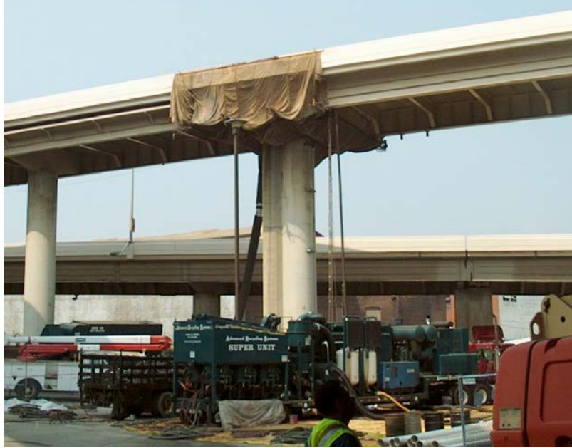
Figure 3.15 Containment Structure Attached to Girder Ends.
