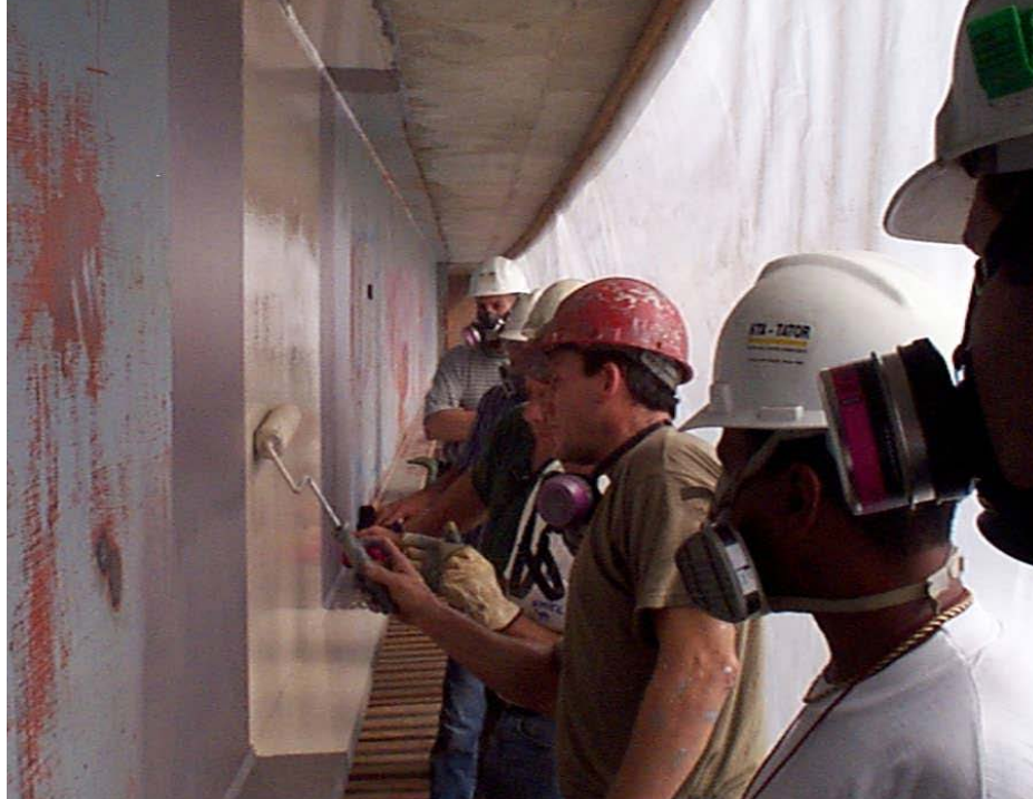
Figure 3.21 Paint Application Using a Roller
