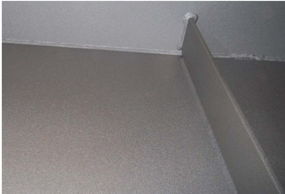
Figure 3.8 Girder Cleaned to the SSPC-SP 10/NACE No. 2 Standard This approach is commonly used on remove-and-replace projects with zinc-based primers.
