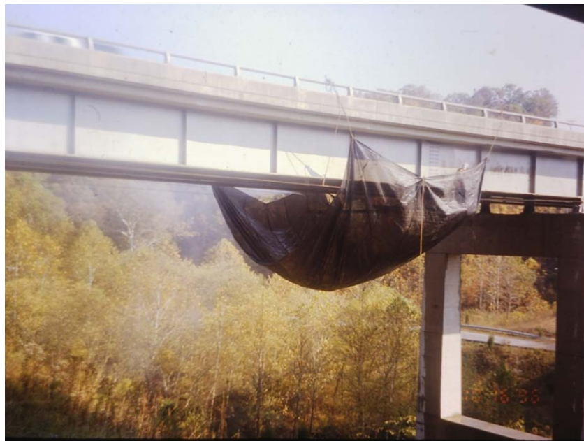
Figure 3.16 Permeable Tarp Diaper
