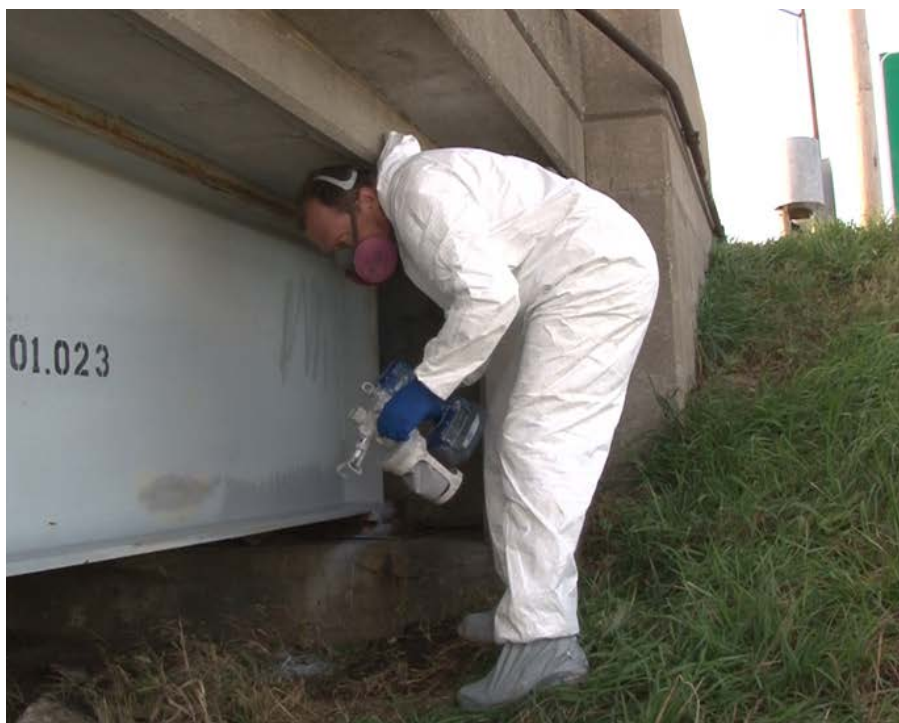
Figure 4.11 Spot Repair Spray Painting Using a Portable Spray Gun
