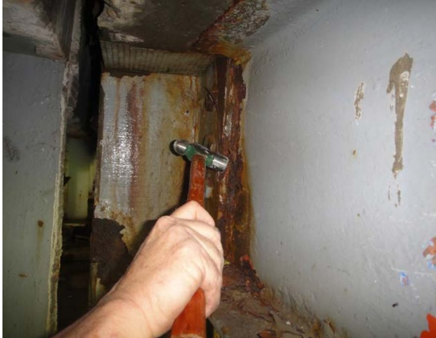
Figure 3.1 Removal of Stratified Rust and Pack Rust with a Hammer Rust is found between riveted steel members.
