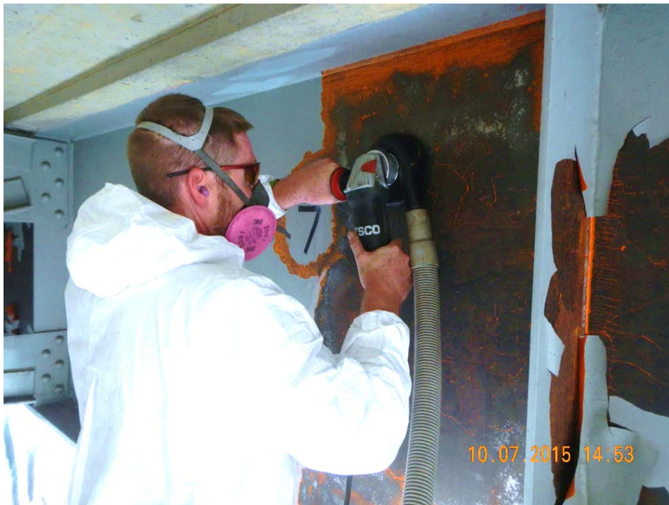
Figure 3.4 SSPC-SP 3 Power Tool Cleaning
