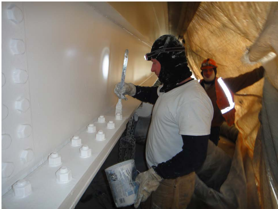
Figure 3.20 Brush Application of Primer on Bolts
