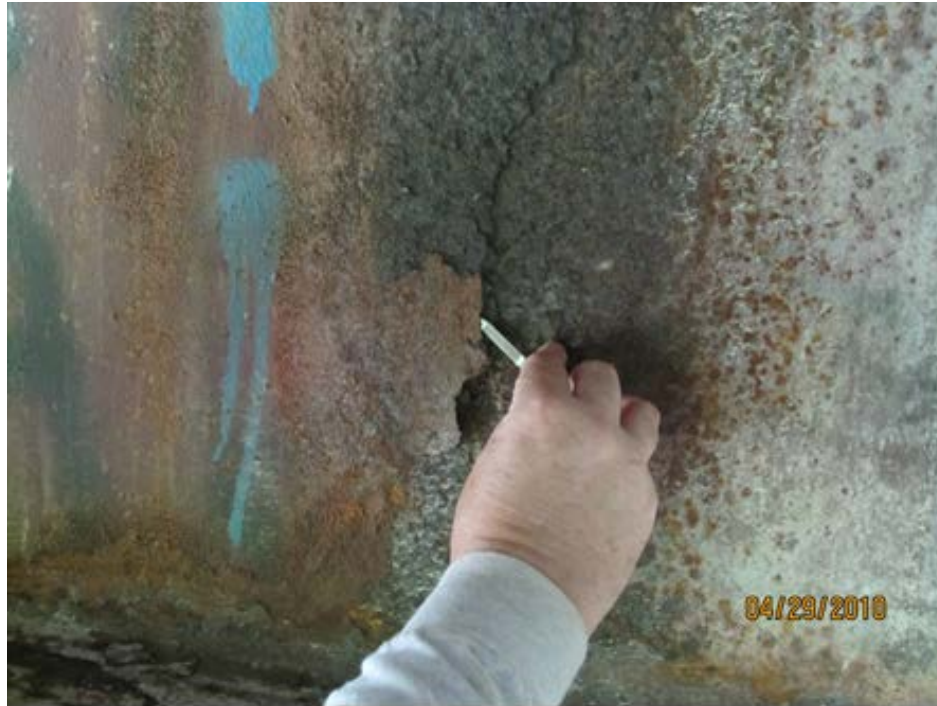
Figure 1.7 Surface Scaling Rust of a UWS Patina on a KYTC Bridge
