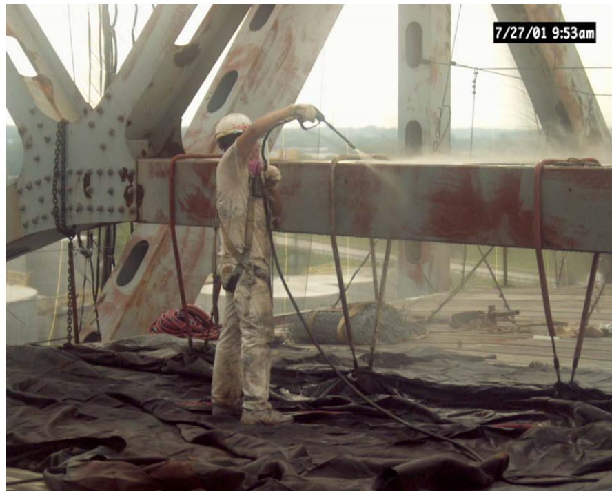
Figure 3.2 Pressure Washing a Steel Member
