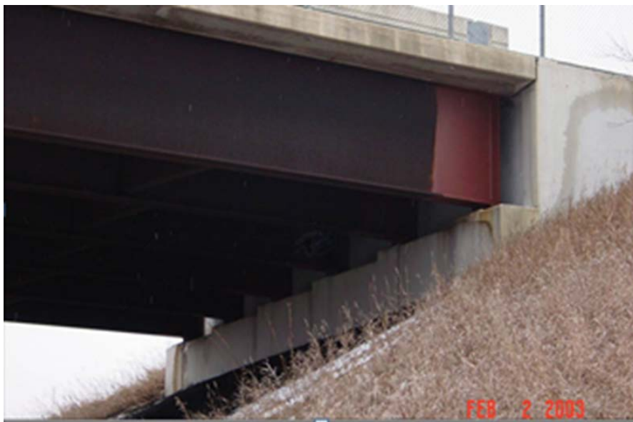
Figure 3.10 Small Zone Painting Repair on a Minnesota DOT UWS Bridge
