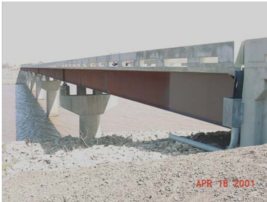
Figure 2.4 Kansas DOT UWS Zone-Painted Bridge Note the area about 20 feet wide from girder end.
