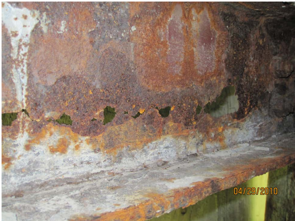
Figure 1.2 Web Rust-Through of a UWS Diaphragm
