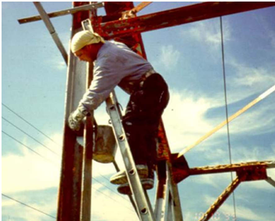
Figure 3.22 Use of Paint Mitt to Apply Coatings
