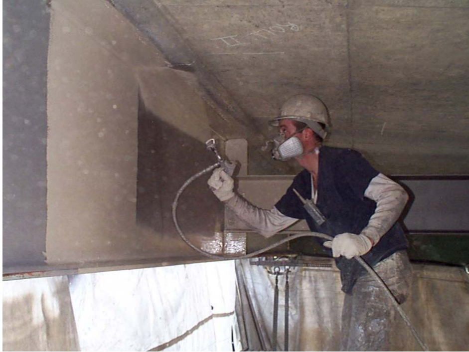
Figure 3.19 Spray Application of a Finish Coat
