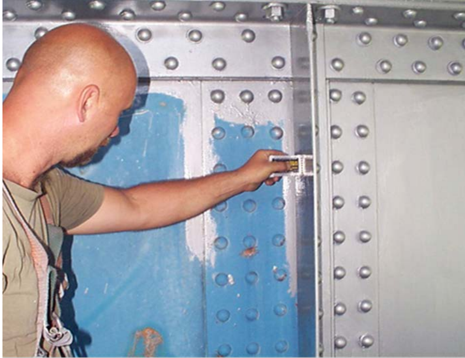
Figure 4.13 Measuring Wet Film Thickness Using a Tooth Gage
