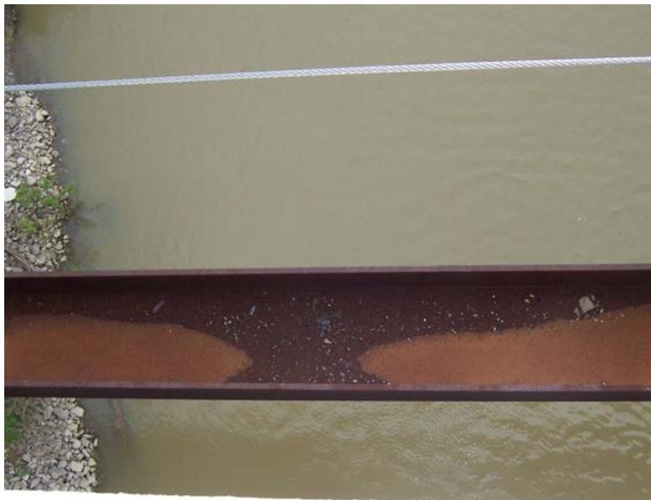
Figure 2.14 H-girder Lower Chord with Problematic Debris and Moisture Buildup
