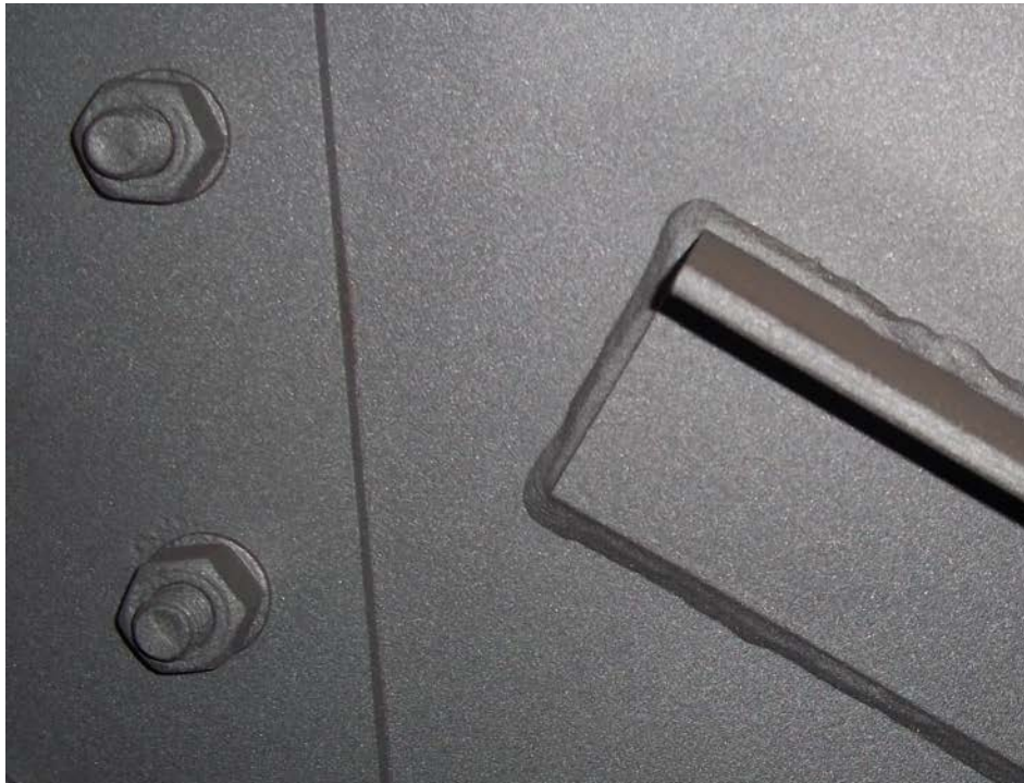
Figure 3.14 Surface Profile of Steel Cleaned to the SSPC-SP 10/NACE No. 2 Standard
