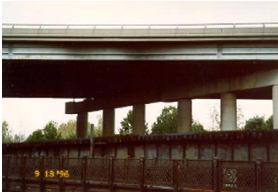
Figure 2.7 Diesel Fume Deposits on Girders of a KYTC Overpass Bridge
