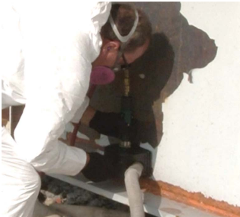
Figure 3.6 SSPC SP-11 Power Tool Cleaning of a Girder
