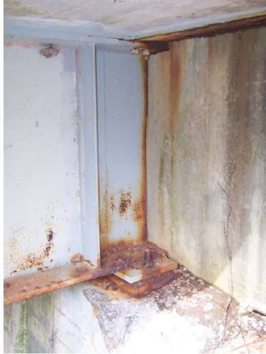
Figure 1.3 Typical Girder/Beam End Corrosion
