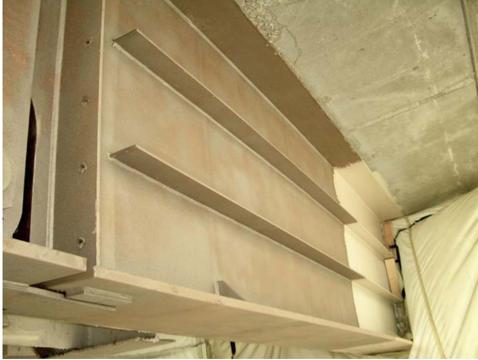
Figure 3.13 Girder Cleaned to the SSPC-SP 14/NACE No. 8 Standard Compare this finish to the one shown in Figure 3.8.
