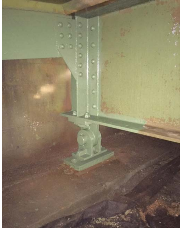
Figure 2.1 Spot Coating Applied to a Beam End, Diaphragm, and Bearing
