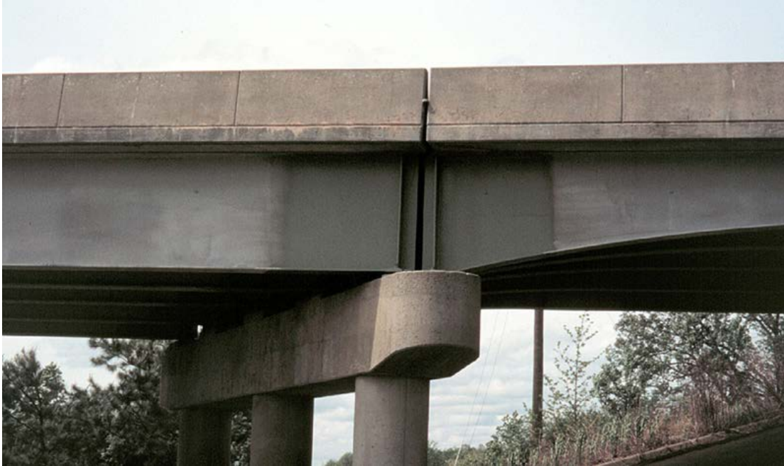
Figure 2.3 Zone Painting on Beam Ends of a KYTC Overpass Bridge New paint was used to repair coating damage due to joint leakage above the beams.
