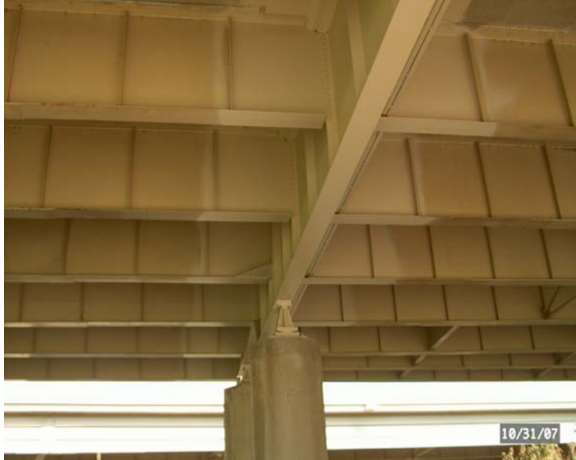
Figure 2.5 Color Matching on a Zone Painting Project The project involved girder ends and floor beams under deck joints.
