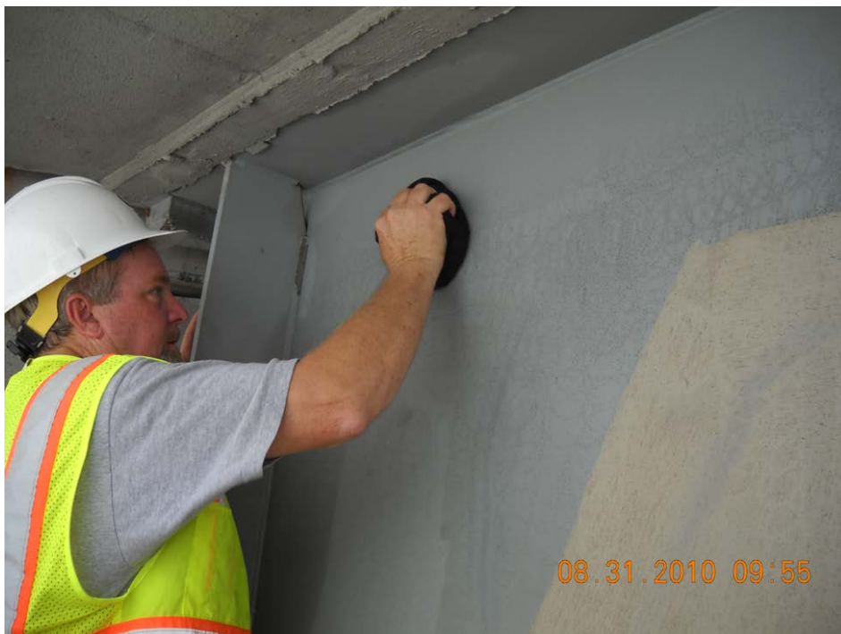
Figure 4.6 Inspector Wiping a Prepared Surface
