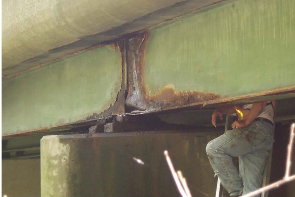
Figure 1.1 Web Crippling of a Girder
