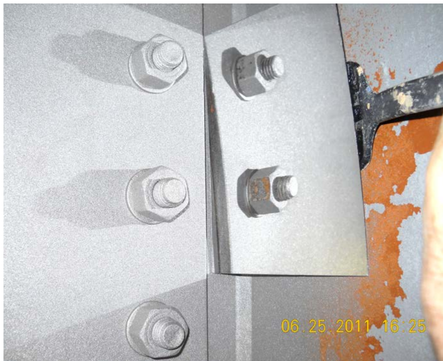
Figure 4.8 Mirror Inspection of Hex Nuts This technique is used by inspectors to detect locations incompletely cleaned by abrasive blasting.
