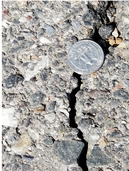
(a) Crack width less than 1/2 inch
