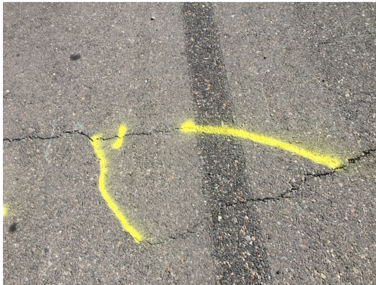
(c) Block cracks in Number 9
