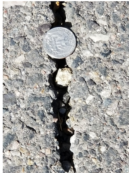
(b) Crack width more than 1/2 inch
