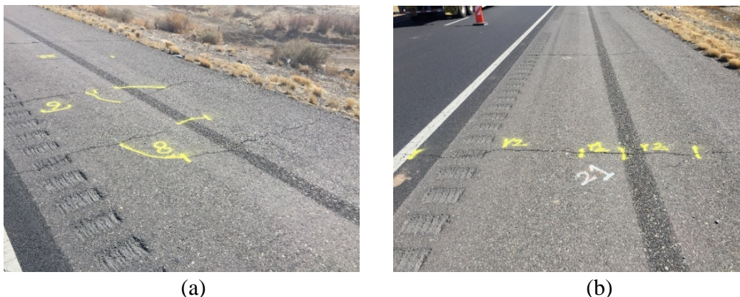
FIGURE 32 Transverse Cracks on I-40 instrumentation section
