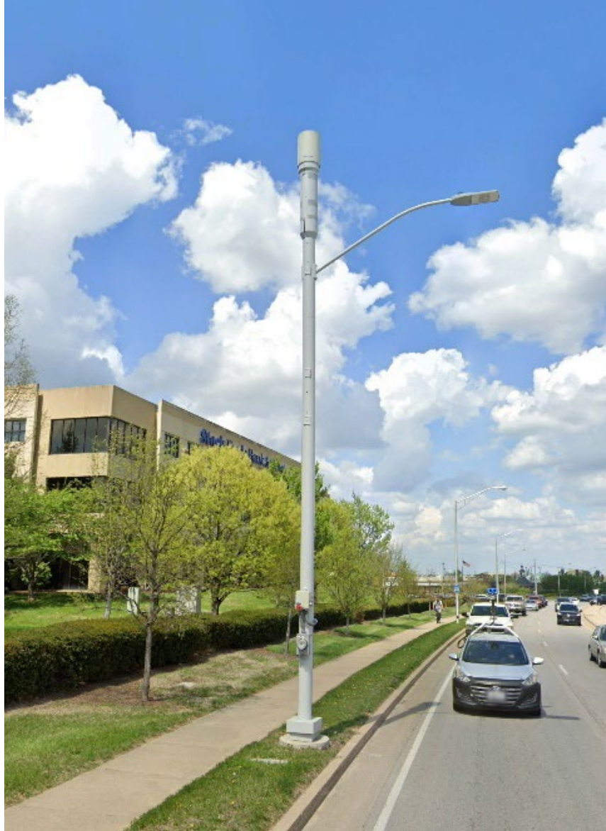
Figure 3.16 Small Cell Wireless on Light Pole in Lexington, Kentucky
