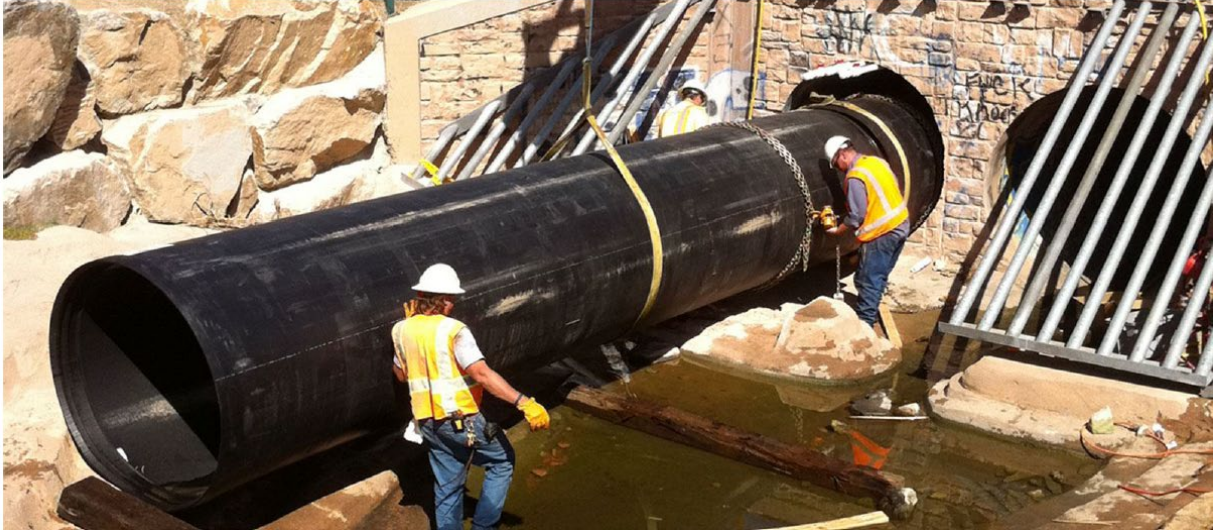
FIGURE 3 Culvert retrofit using HDPE pipes [2].
