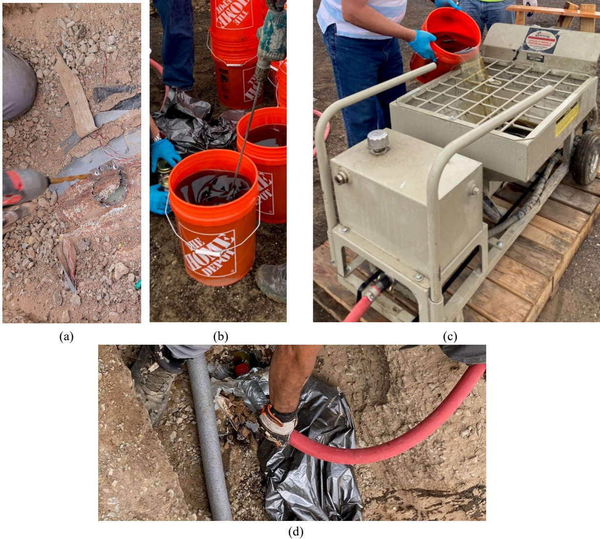
FIGURE 22 Mixing and pumping polymer in the annular space using an opening at the middle of the span. (a) perforation to inject polymer. (b) polymer mixing. (c) polymer pumping. (d) polymer injection.
