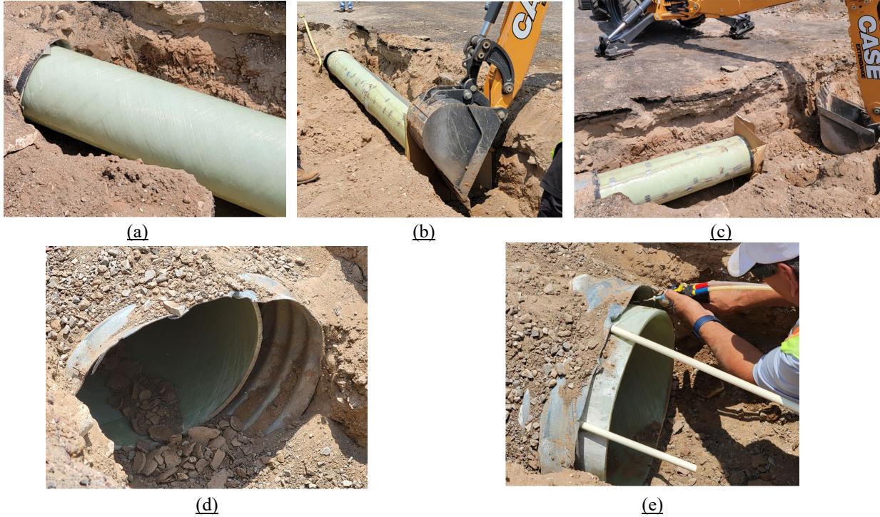
FIGURE 20 (a)-(c) Slip-Lining Process driving the GFRP pipe inside the corrugated metal culvert. (d)-(e) GFRP pipe completely slid inside the corrugated metal culvert and application of the closure foam prior to grouting of the annular space.
