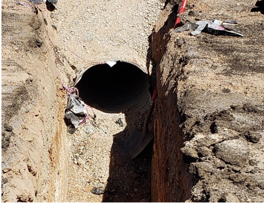
FIGURE 12 Buried corroded metal pipe
