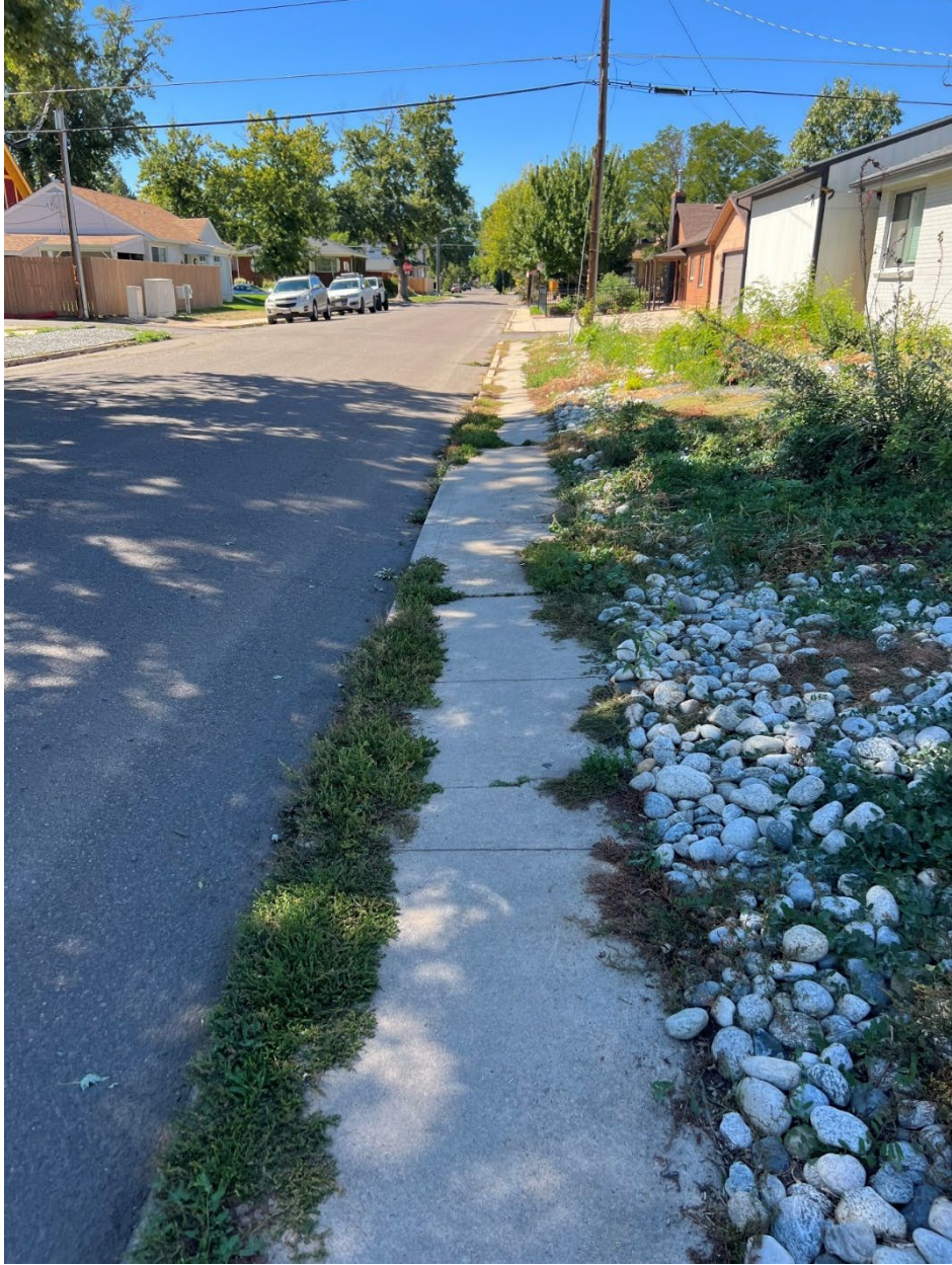
Figure 3.8 28 th Avenue Sidewalk
