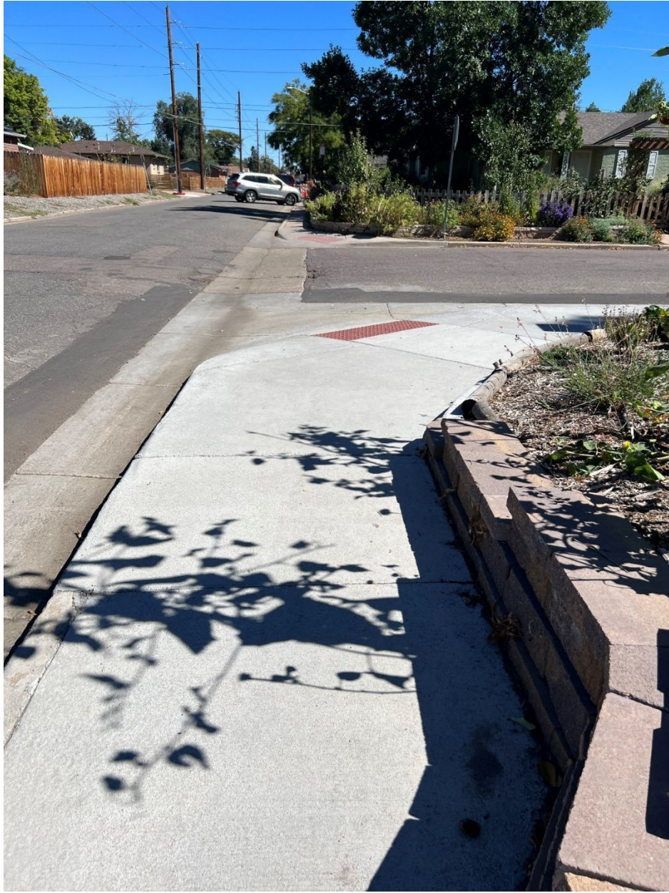
Figure 3.5 29 th Avenue and Elm Street Curb Ramp
