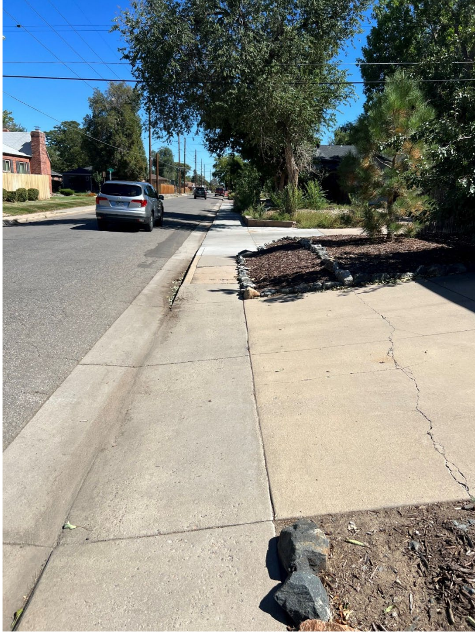
Figure 3.9 29 th Avenue Sidewalk
