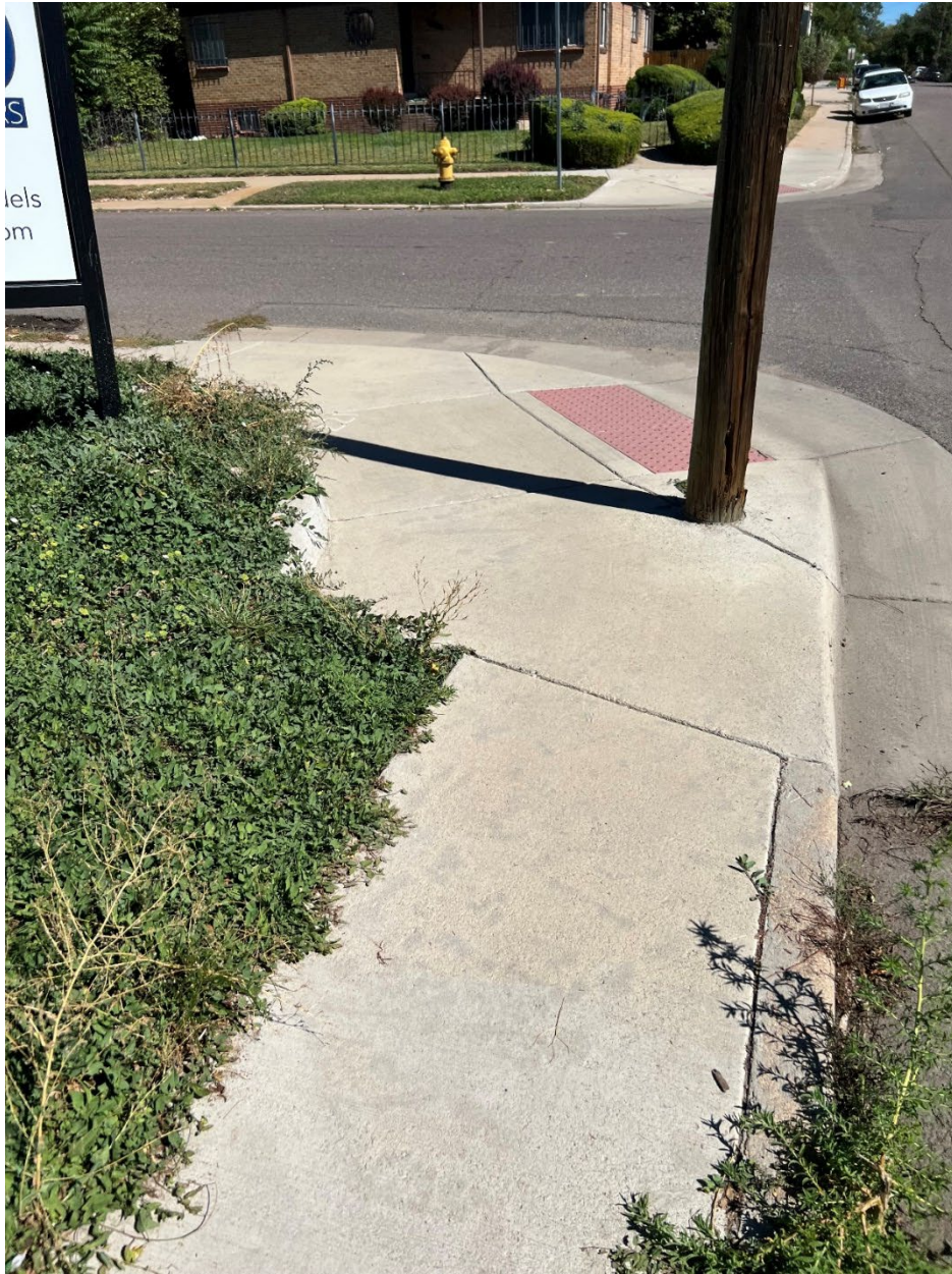
Figure 3.3 28 th Avenue and Elm Street Curb Ramp
