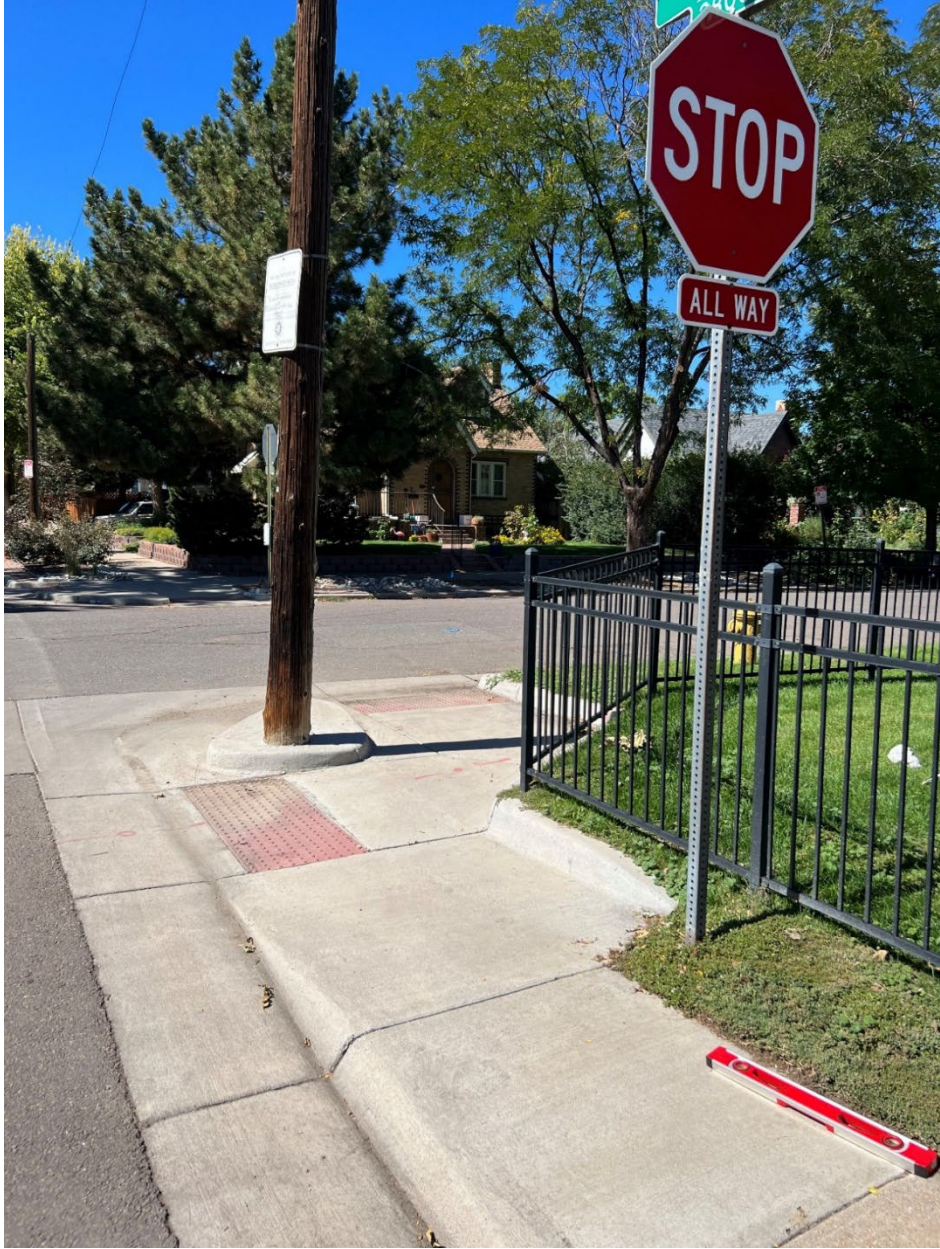
Figure 3.4 28 th Avenue and Eudora Street Curb Ramp
