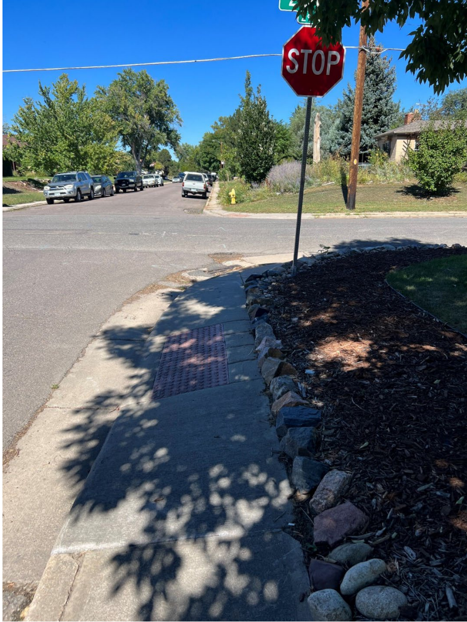
Figure 3.6 29 th Avenue and Eudora Street Curb Ramp
