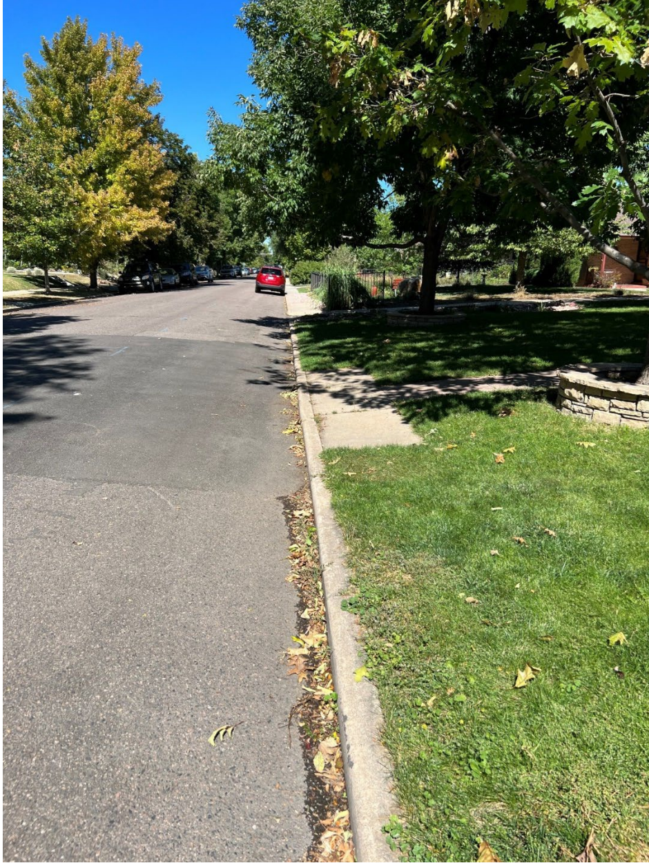
Figure 3.11 Eudora Street Sidewalk
