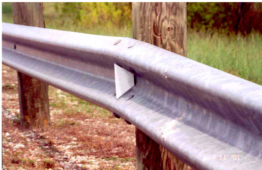
Figure 5-26. Reflector Installed in Guardrail.
