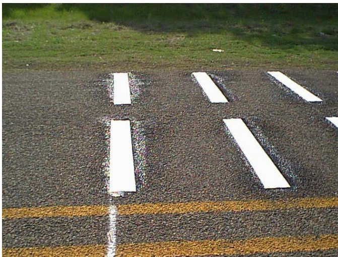
Figure 7-25. Recently Replaced Rumble Strips.
