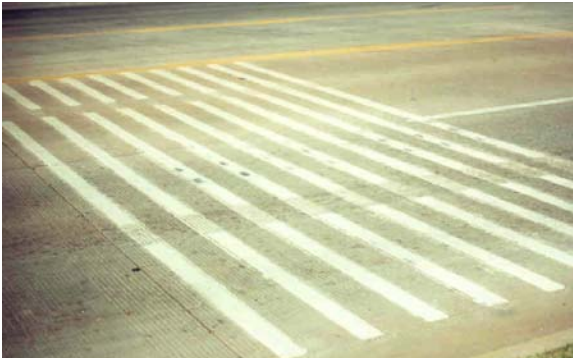
Figure 6-6. Example of Full-Width Approach Rumble Strips.
