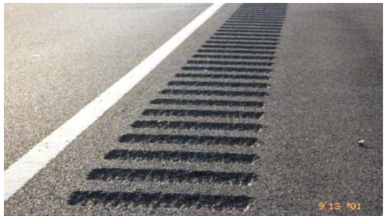
Figure 7-17. Close-Up of Edge Line Rumble Strips.
