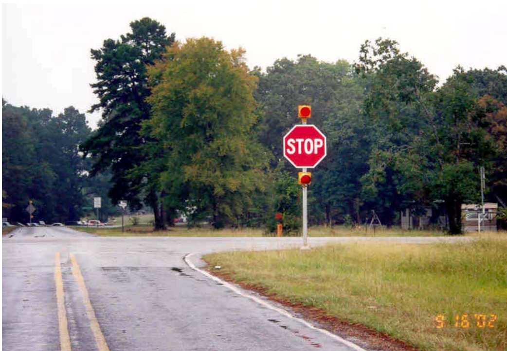
Figure 6-5. Example of Stop Sign with Flashers.
