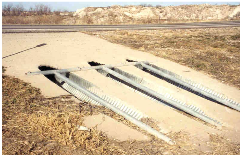
Figure 7-10. New Safety End Treatment on FM 1212.
