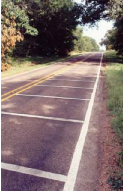
Figure 7-12. Rumble Strips Warning of Approaching Intersection.
