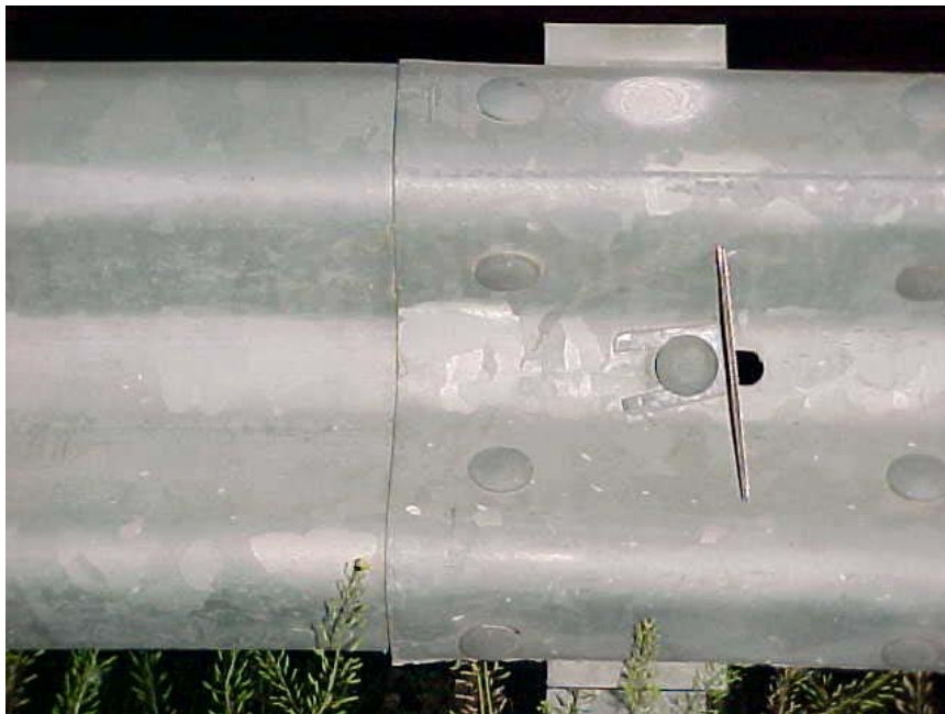
Figure 7-4. Close-Up of Barrier Reflector.
