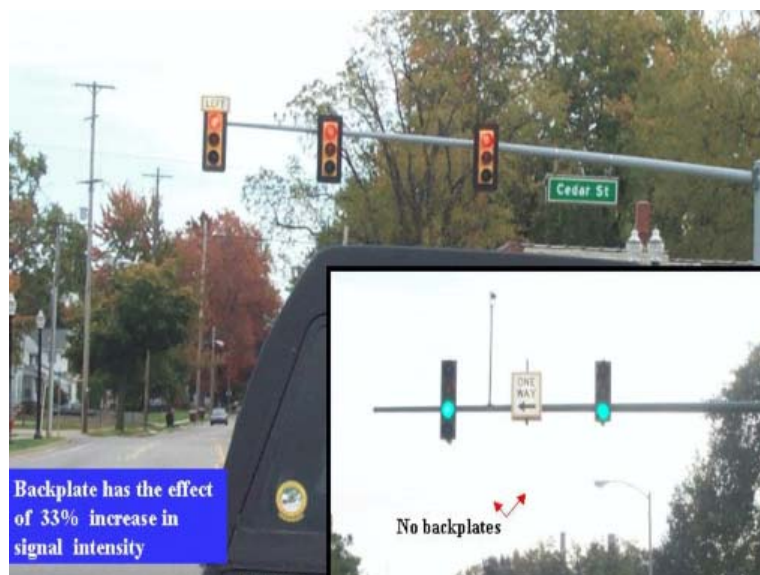
Figure 6-15. Heads with and without Backplates (111).
