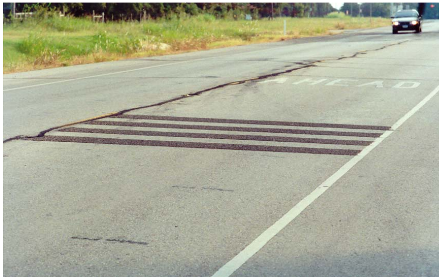
Figure 7-43. Rumble Strips and Pavement Markings on FM 1179.
