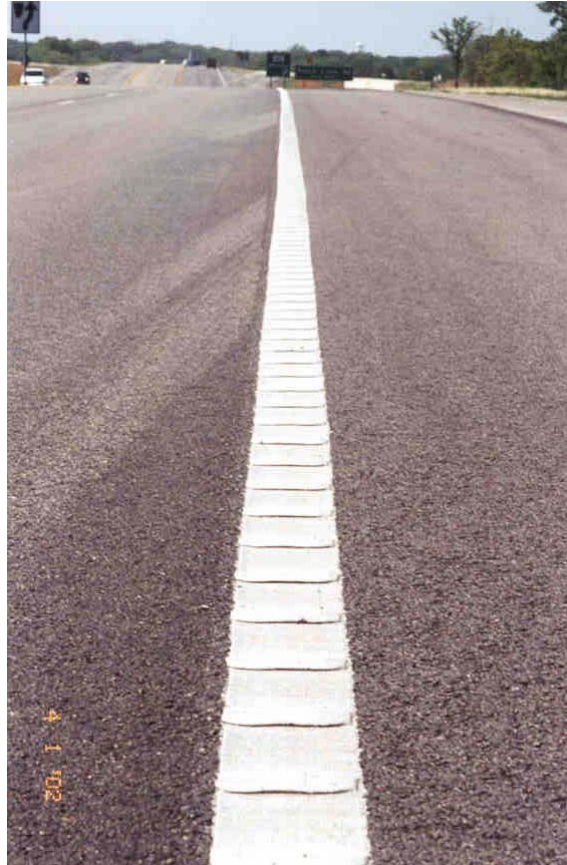
Figure 7-36. Edge Line Profile Markings.
