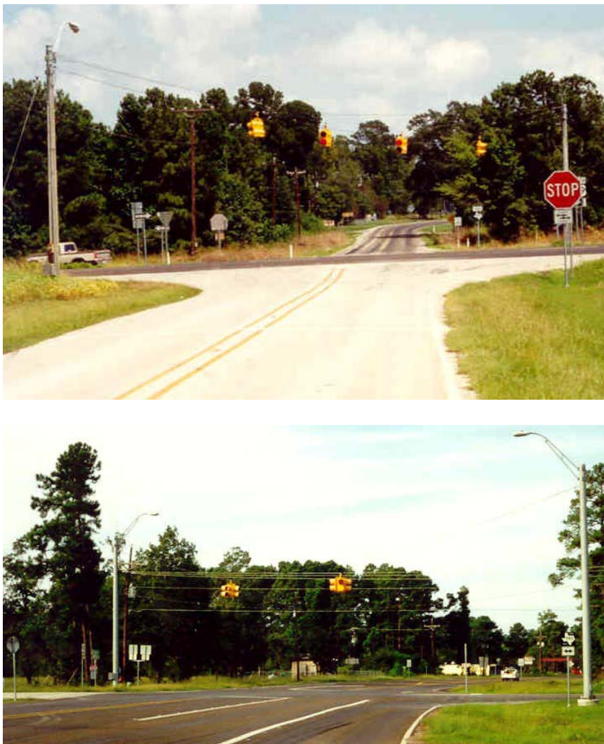
Figure 6-11. Examples of Intersections with Flashing Beacons.
