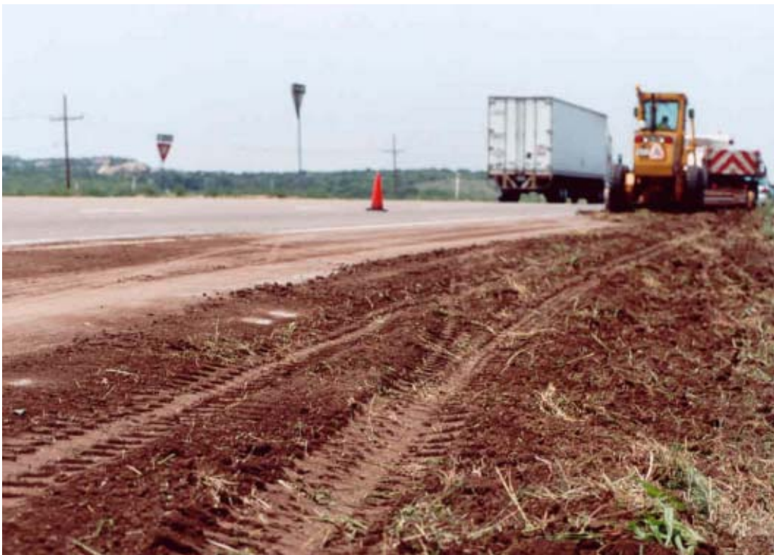
Figure 7-31. Motor Grader Adding Fill Material to Shoulder.
