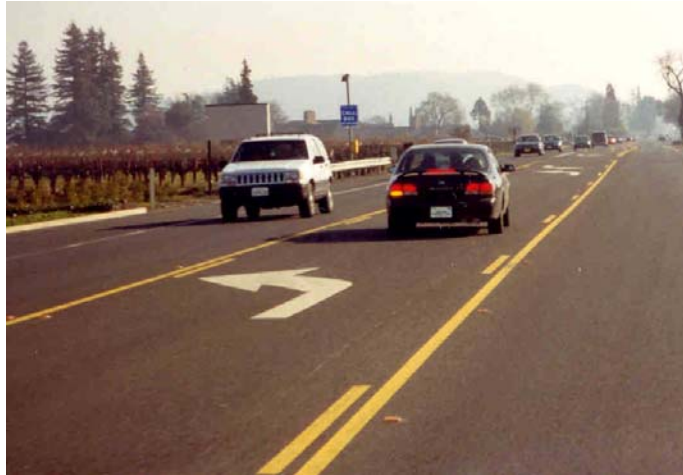
Figure 5-6. Example of Two-Way Left-Turn Lane in Rural Area (2).
