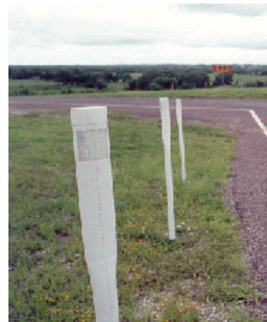
Figure 5-24. Example of Post-Mounted Delineator.
