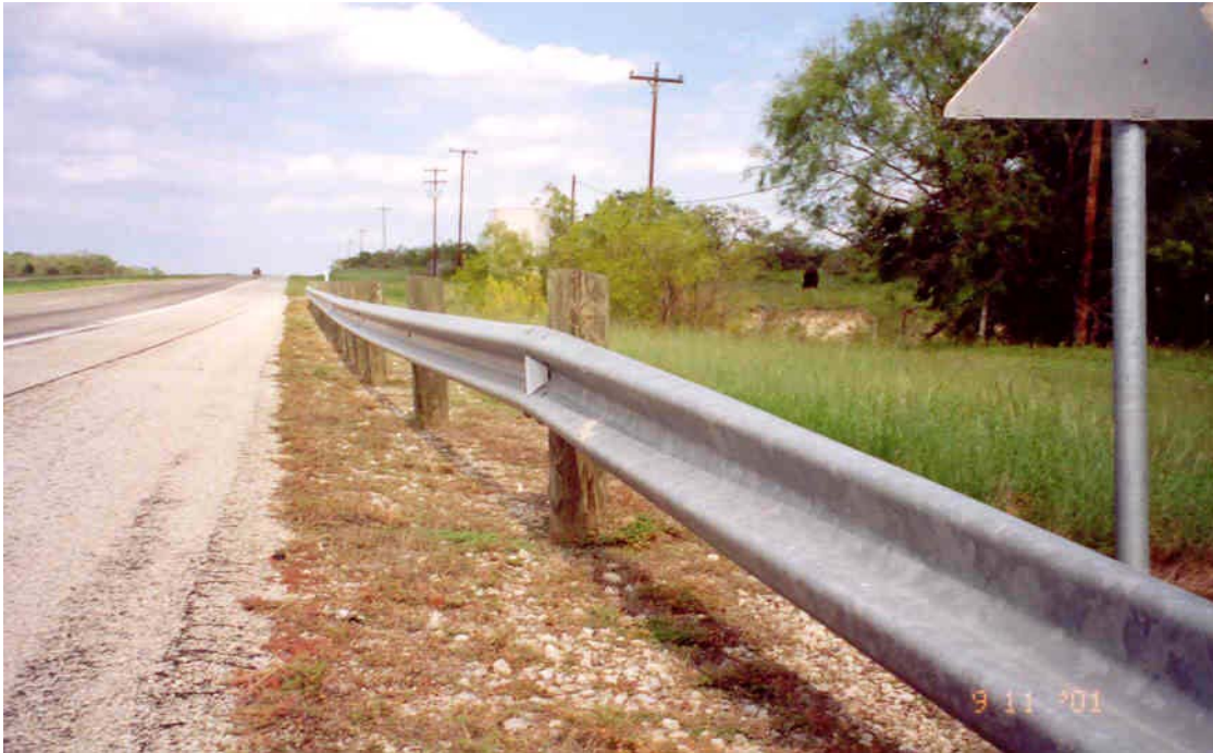
Figure 5-27. Two-Lane Highway with Barrier Reflectors.
