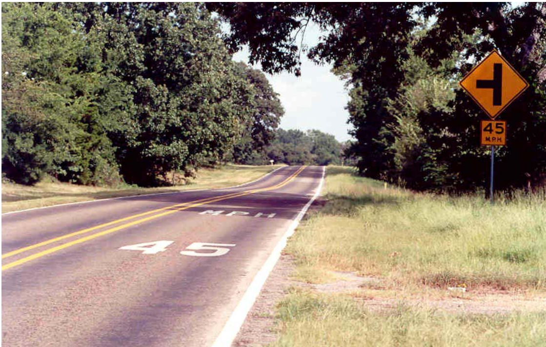
Figure 7-13. Pavement Markings Supplementing Advisory Speed Sign.
