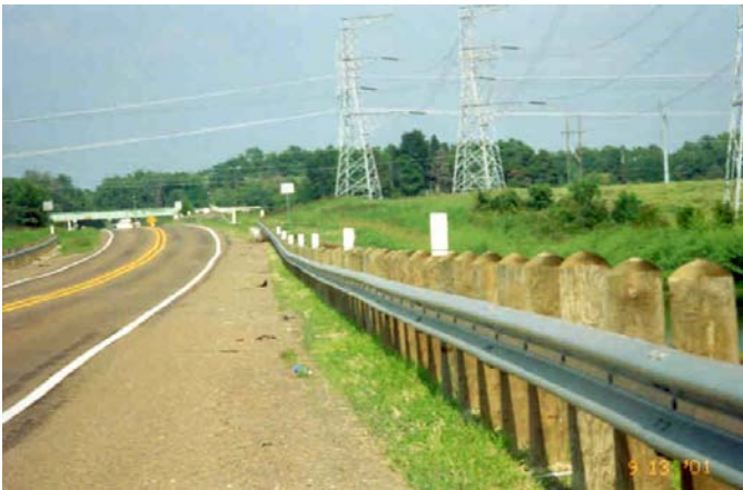
Figure 5-25. Post-Mounted Delineators with a Guard Rail.
