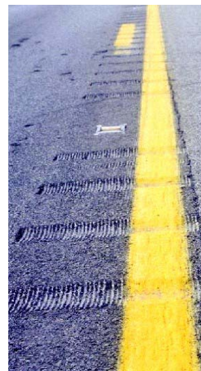
Figure 5-3. Examples of Centerline Rumble Strips.
