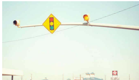
Figure 6-1. Example of Overhead Advance Signing.
