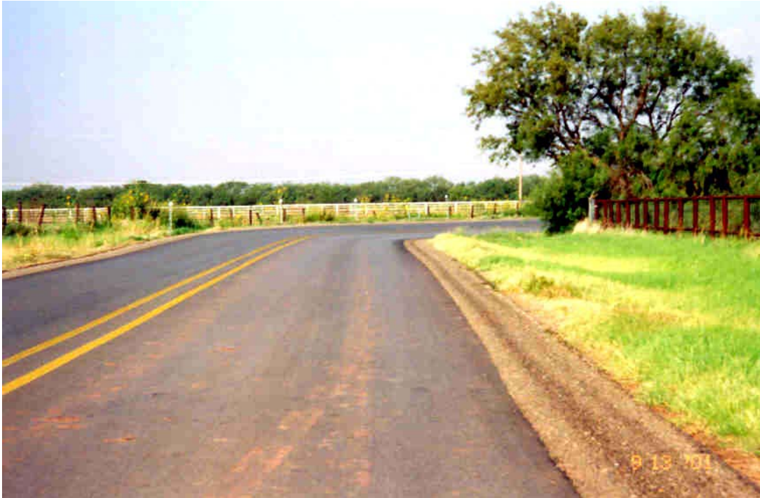
Figure 5-11. Example of Centerline Only Pavement Markings.
