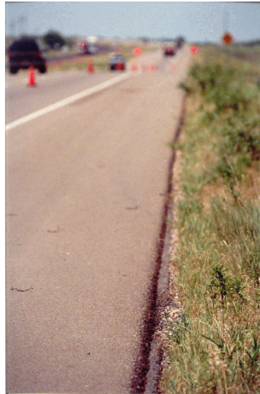
Figure 5-9. Shoulder Drop-Off.
