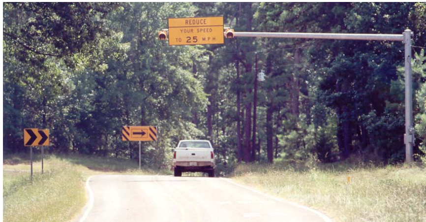
Figure 7-23. Various Warning Devices for Horizontal Curve.
