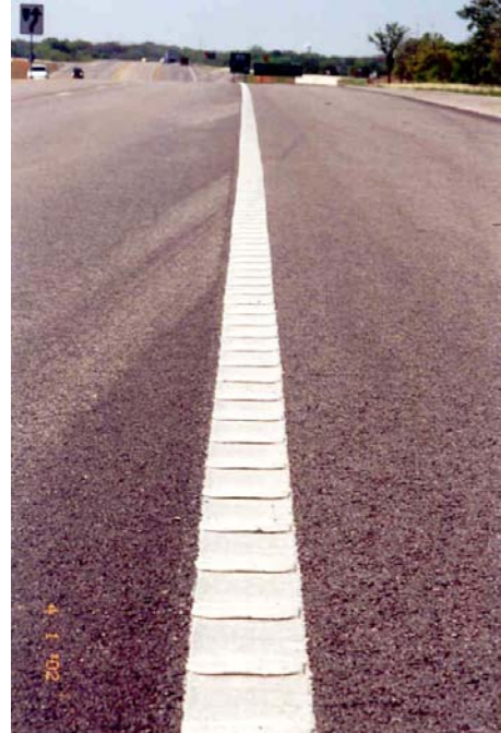
Figure 5-2. Examples of Thermoplastic Profile Markings.
