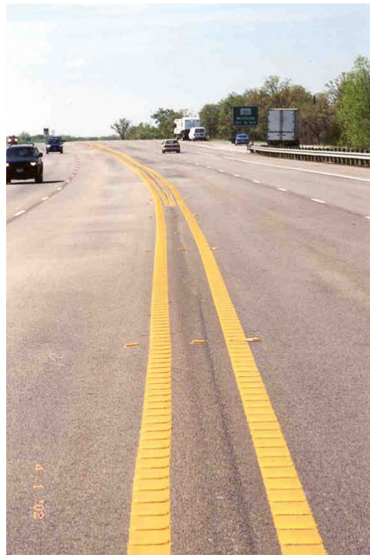
Figure 7-35. Centerline Profile Markings.
