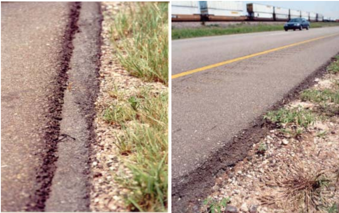
Figure 7-30. Shoulder Drop-Off Examples.
