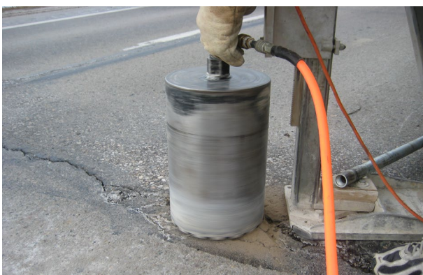
Coring operation performed with 254 mm drill bit using air as drilling medium
