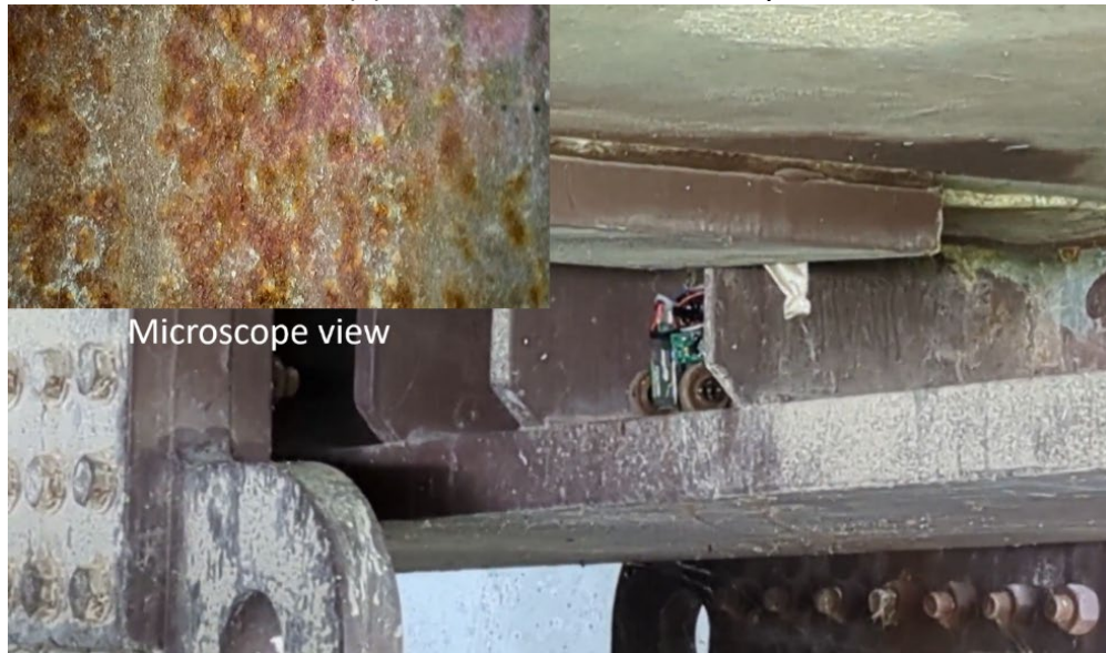
(b) Transverse stiffeners at the end of steel girder
