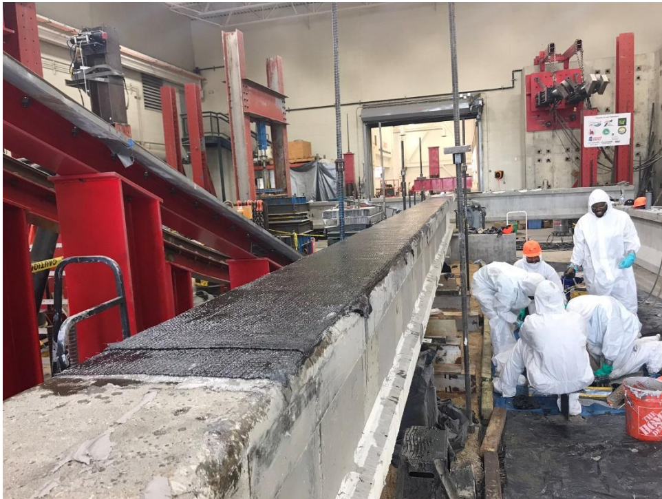
Figure G-23. CFRP wet layup system application to the girder
