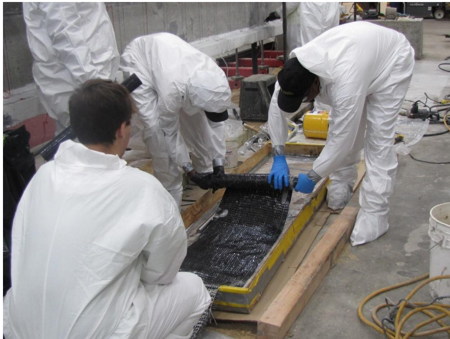
Figure G-18. Wet layup system of CFRP preparation of the repaired girder
