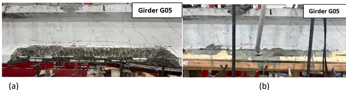
Figure 6-13. Girder G05 with 33% strand damage (a) Strand splicing configuration, (b) Formwork used for splicing repair
