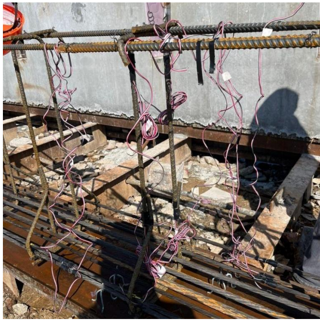
Figure B-32. Installing strain gages at the girder fabrication phase
