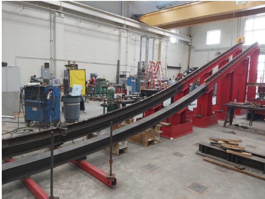
Figure B-27. Completing installing the curved supporting beams from two sides
