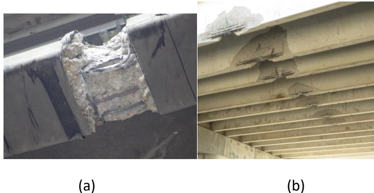
Figure A-11. Photographs of over-height vehicle collisions with bridge prestressed girders (a) Galloway road over I-84 (Courtesy of IDAHO DOT), and (b) Bridge over US 50 East (Courtesy of Missouri DOT)
