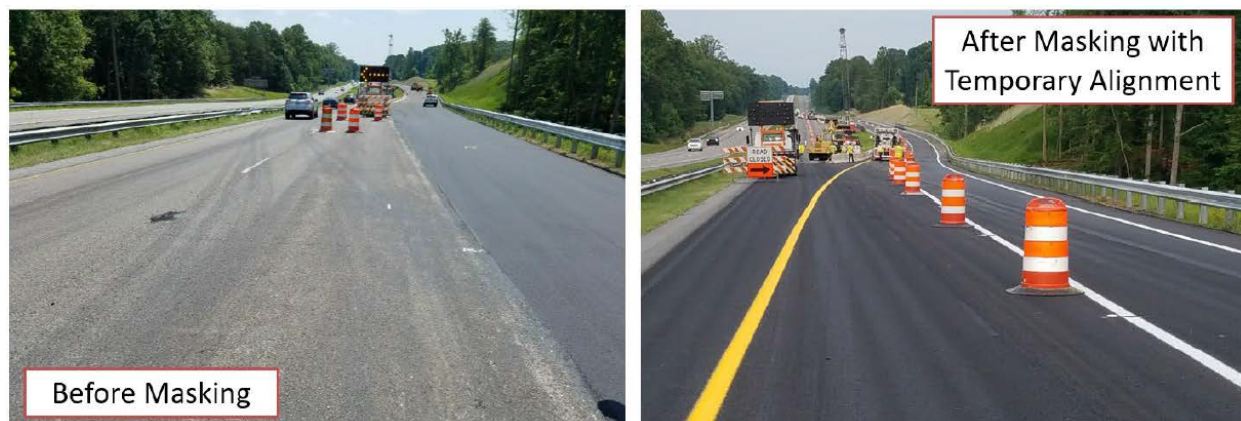
Figure 19. Example of Painting Pavement Surface Black during Work Activity [260]
