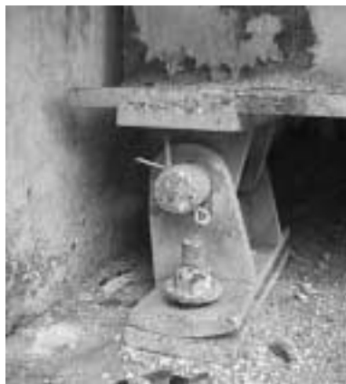
Figure 1.3: A rocker support at an abutment
