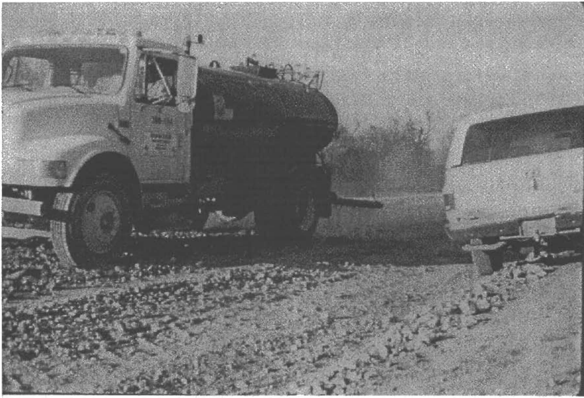
Figure 5.13: Addition of Water Prior to Compaction.
