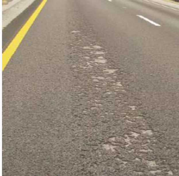
FIGURE 6 Raveling problem associated with OGFC (7)
