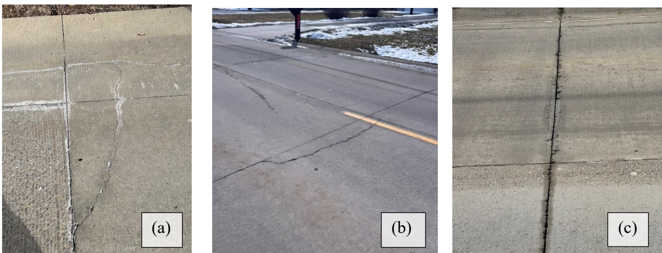
Figure 14. Photo. Types of distresses observed on East Grand Road: (a) corner cracks, (b) transverse crack parallel to transverse joint, and (c) raveling on transverse joint.
