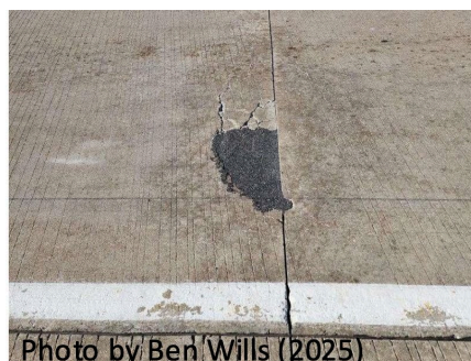
Figure 16. Photo. Distresses observed on I-57 southbound lane during head-to-head traffic phasing.
