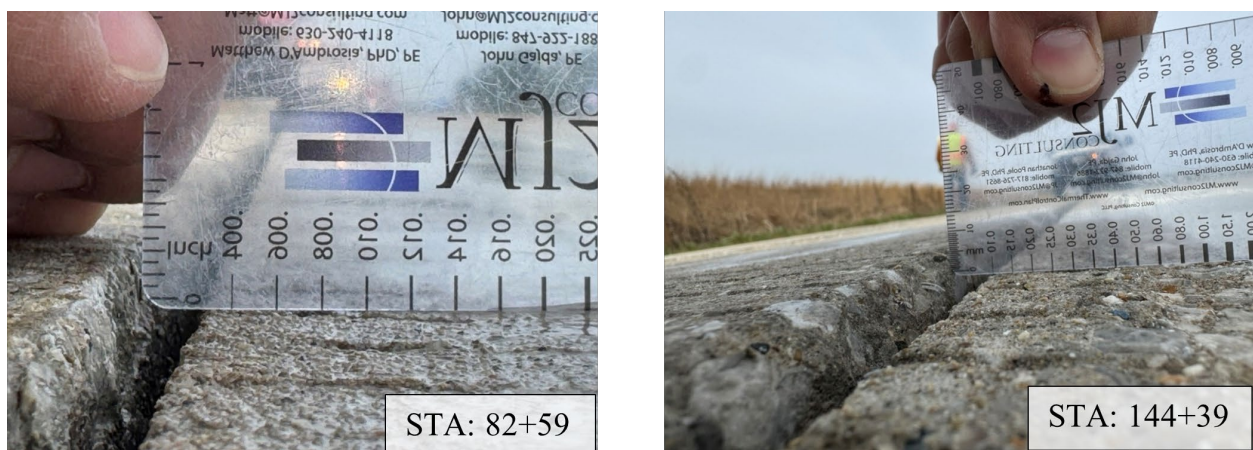
Figure 10. Photo. Example of faulting along driving lane-shoulder joint of 0.25 in. (6 mm) on I-72 EB.
