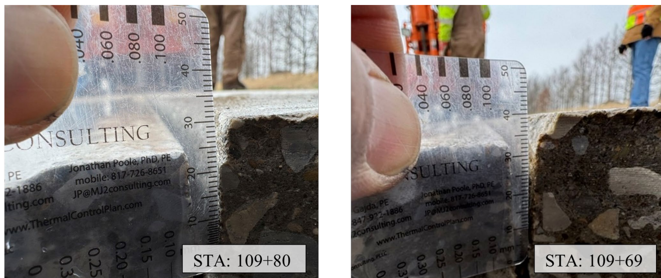
Figure 12. Photo. Faulting along driving lane-shoulder joint at approximately 0.25 in. (6 mm) on I-72 WB.
