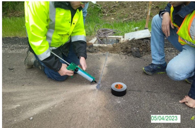
Figure 39 Installation of thermocouples
