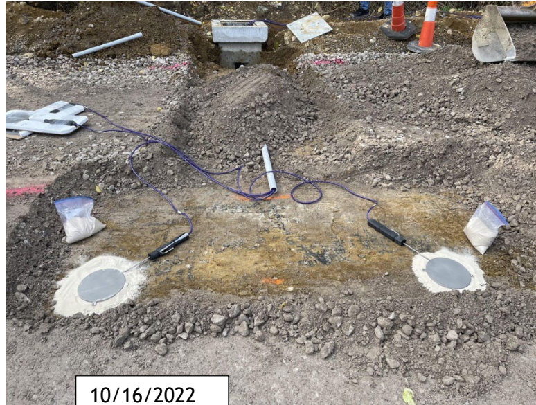
Figure 33 Pressure Cell Installation
