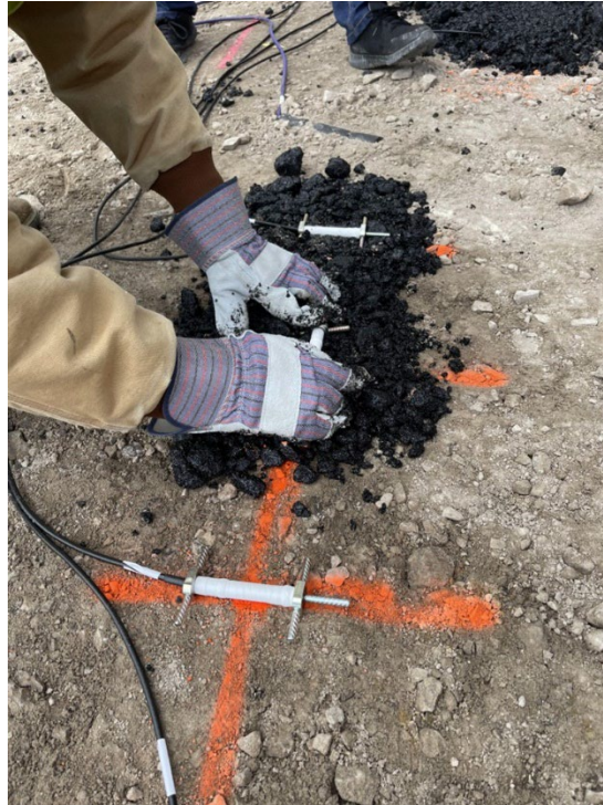
Figure 37 Protecting Strain Gages Prior to Paving
