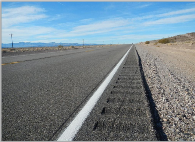
US 95, South of Goldfield: Rumble strips placed within a narrow shoulder make the shoulder unusable for bicyclists.
