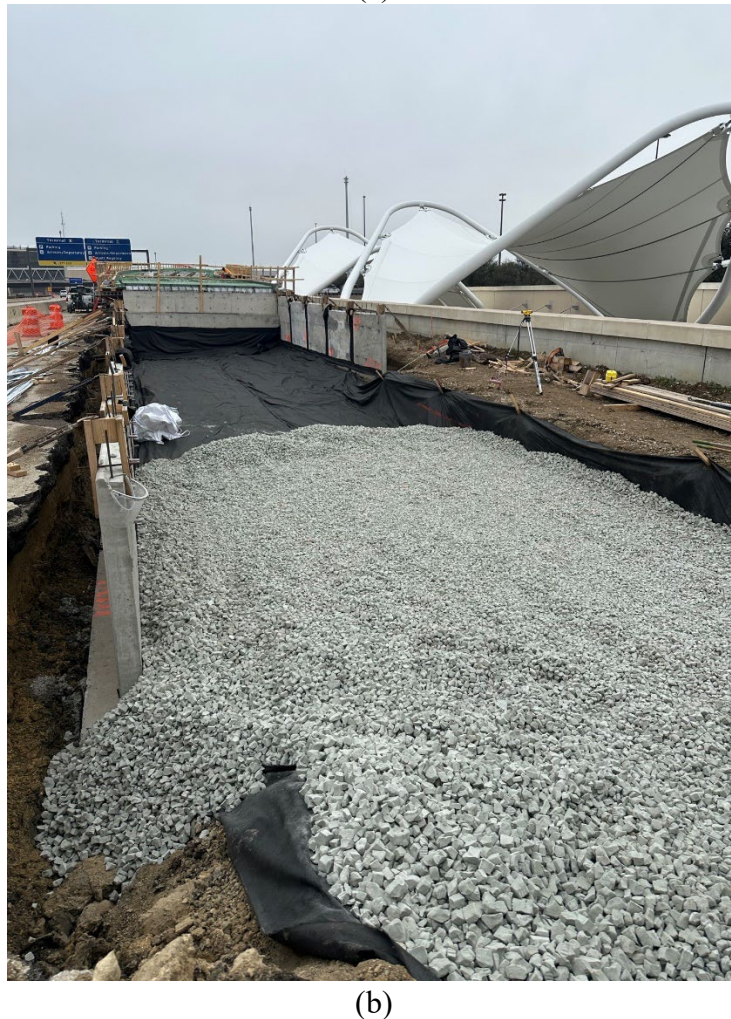
Figure 3.3. (a) Typical cross-section of walls (redrawn from interim review drawings courtesy of AeroAggregates); and (b) photo of MSE walls during construction (courtesy of John Ratiu of AeroAggregates).
