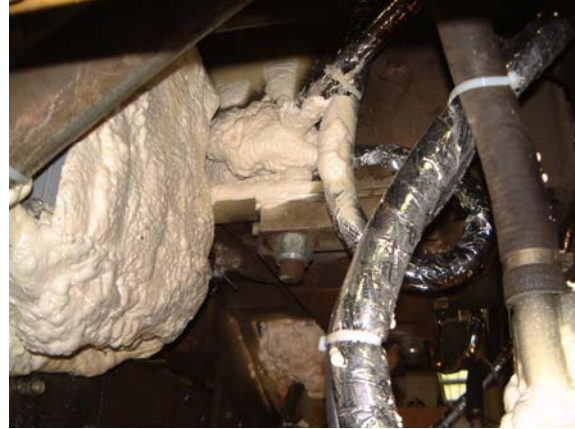
Figure 30: Insulated Metering Box & Insulated/Heat Traced Product Lines
