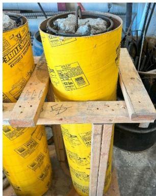
Figure 4.19 Supportive skeleton for the form work
