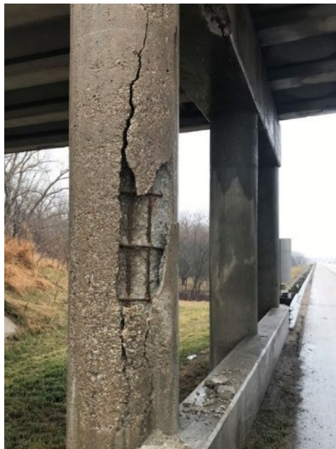
Figure 3.11 Deteriorated bridge column considered in this example
