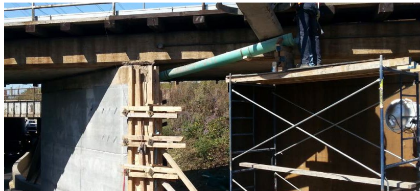
Figure 2.1 Casting UHPC using a chute for a thin jacket for a bridge pier from the top of formwork (Doiron, 2017)
