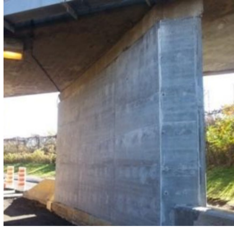
Figure 2.2 UHPC jacket over the bridge pier (Doiron, 2017)
