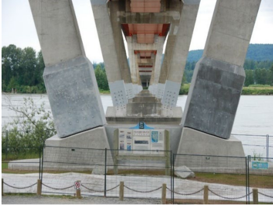
Figure 2.3 Seismic strengthening with UHPC jackets around bridge piers (Doiron, 2017)
