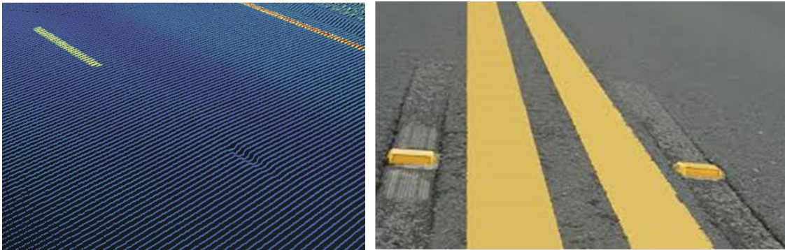
Figure 2.6: Examples of slotted skip pavement markings
