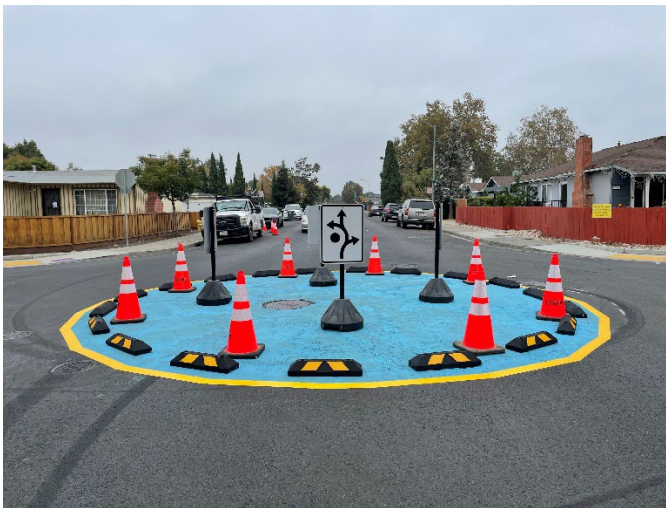
Photo 2: temporary roundabout/traffic circle to slow down traffic and improve traffic flow
