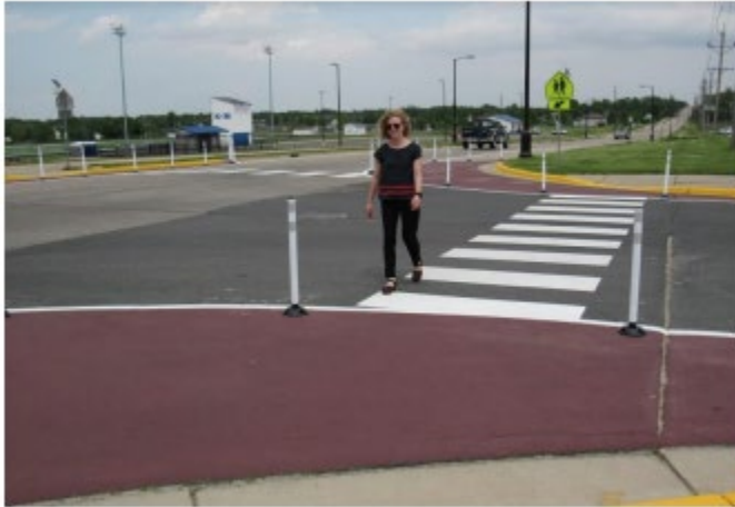
Photo1: extended curb radii with paint and flexible poles that will shorten the crossing distance, make drivers slow down when turning
