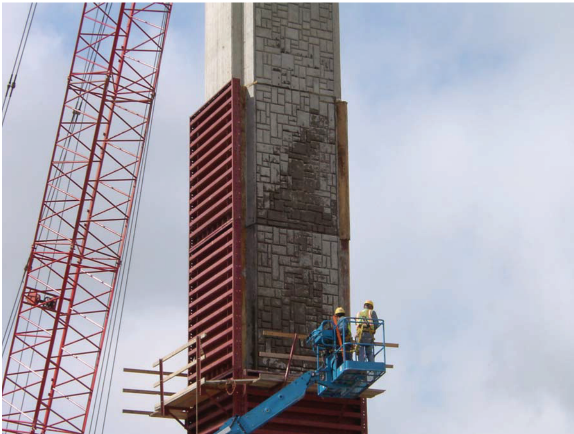
Figure 6 - Rectangular column during form removal and the beginning of construction stage two
