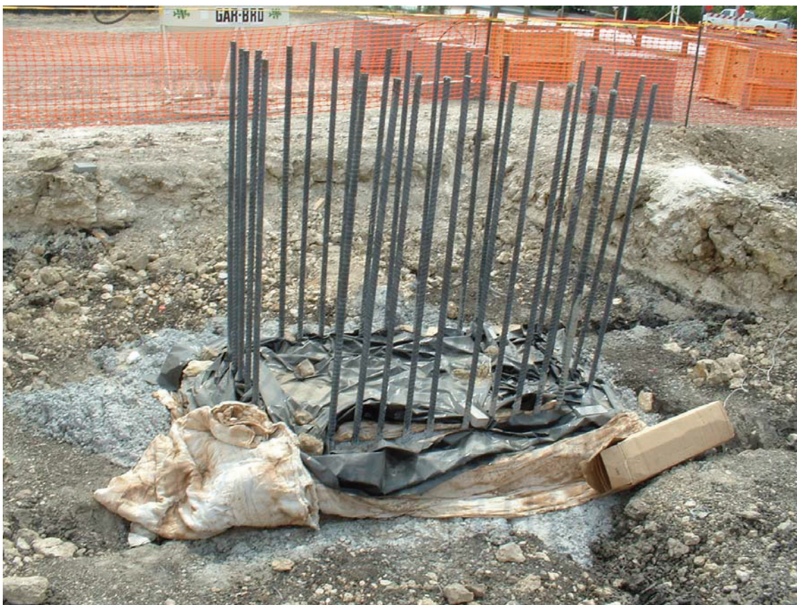
Figure 57 - Example of a footing that would use the Soil on the Sides option
