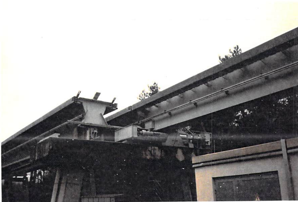
Figure 6. Switch 3 (Two Views)
