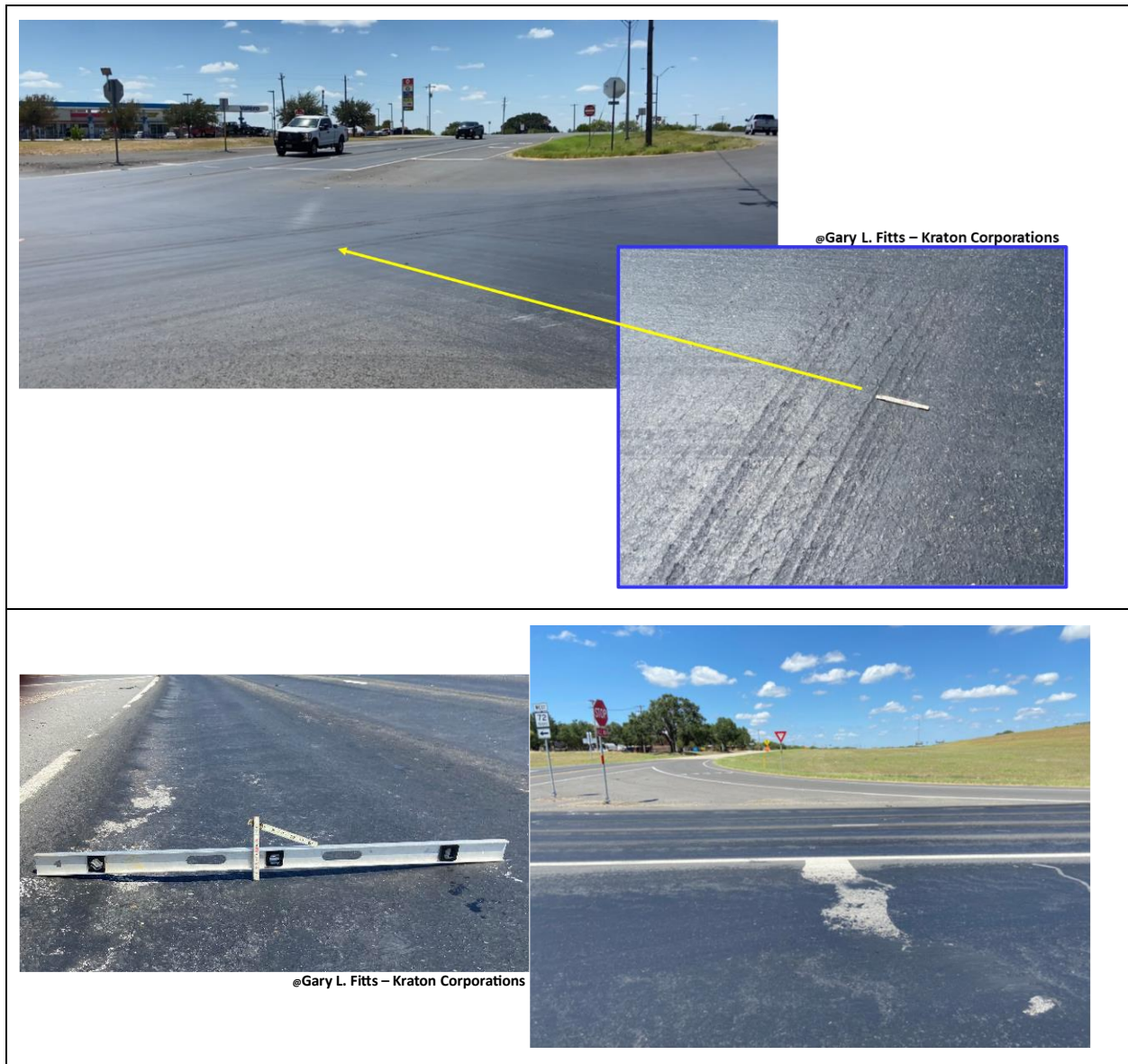
Figure 1-9 Distress like bleeding, rutting and distortion observed in US71 in IH37
