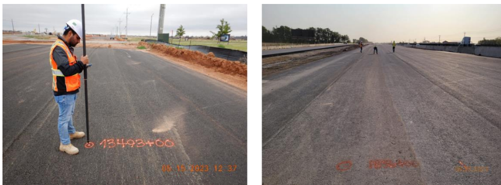
Figure 5-10 Selection of 1000-foot length test section and recording of testing points
