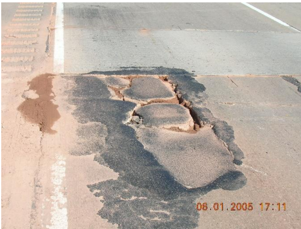
Figure 1-13 Pumping and Punchout in US 287
