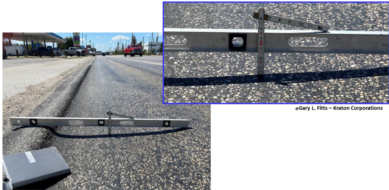
Figure 1-8 Rutting observed in US 281 Intersection
