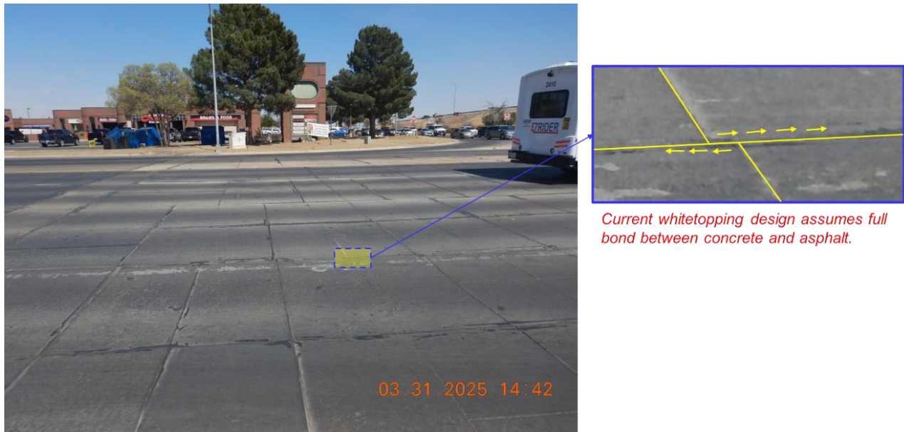
Figure 2-31 Slab Sliding observed in Midland, Texas
