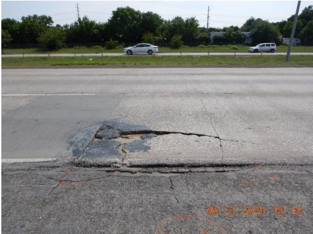
Figure 1-12 Pumping and edge punchout in IH 45
