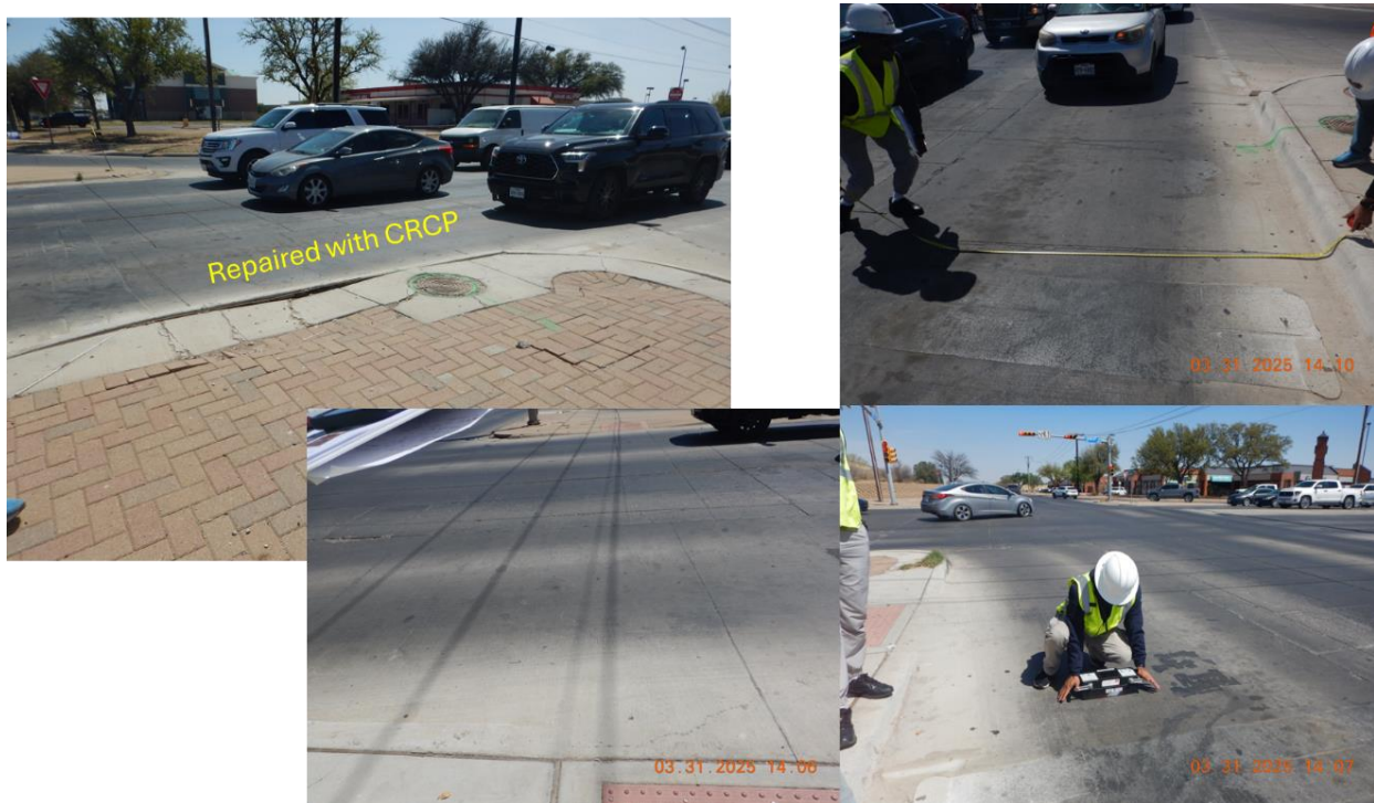
Figure 2-34 Localized distress in CPCD Whitetopping repaired using CRCP
