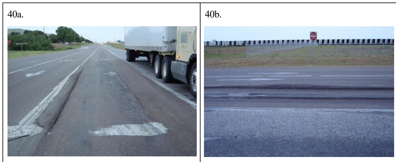
Figure 2-26a. Image of rutting at Intersection 26b. Image of shoving at Intersection
