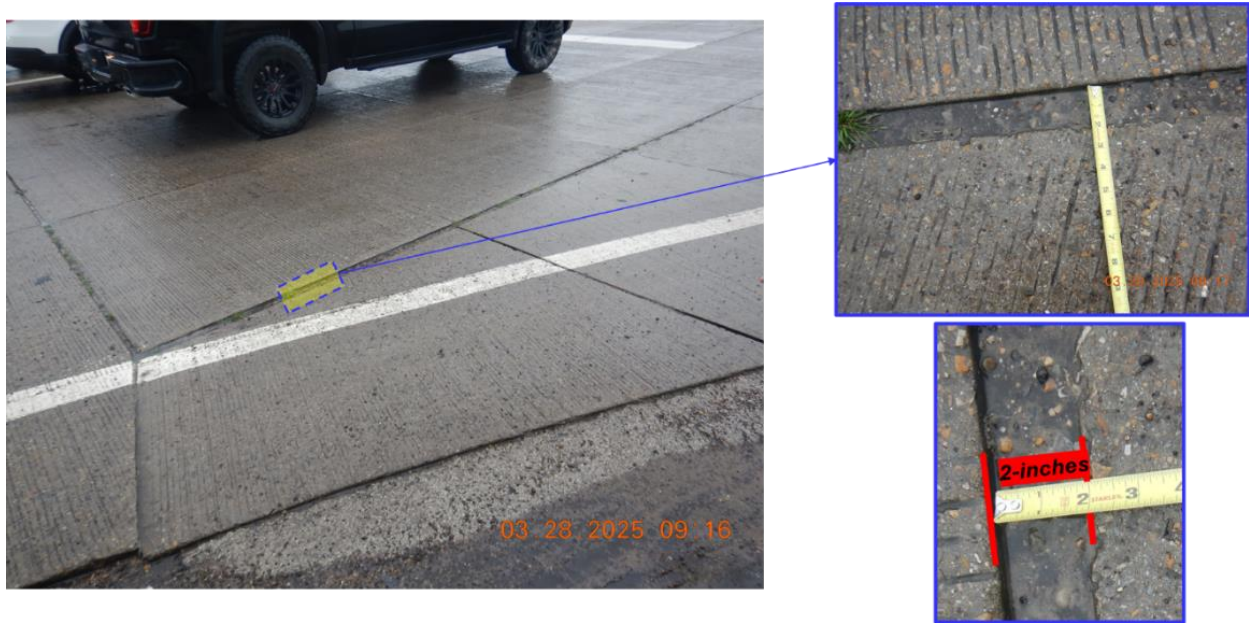
Figure 2-28 Slab Separation of 2-inches observed in Emory, Texas
