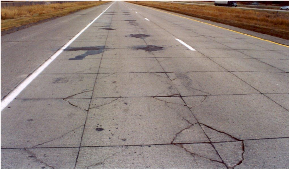
Figure 2-25 Diamond cracking as seen in Minnesota (Burnham, 2005)
