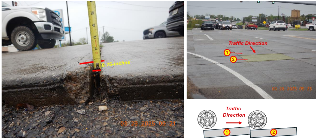
Figure 2-32 Faulting observed in Emory, Texas
