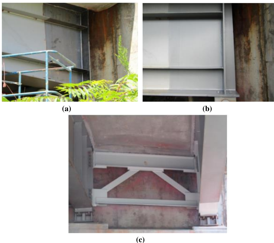
Figure 17. Laser Ablation Coating Removal and Recoating of Route 695 Bridge in August 2017 Showing: (a) After Coating Is Removed on Facia Girder Using Laser Ablation Coating Removal; (b) After Prime Coat Is Applied to Facia Girder No. 4 at Abutment B; (c) After Finish Coat Is Applied to Cross Frame between Girders No. 3 and 4 and to the Bottom of Girder No. 4.
