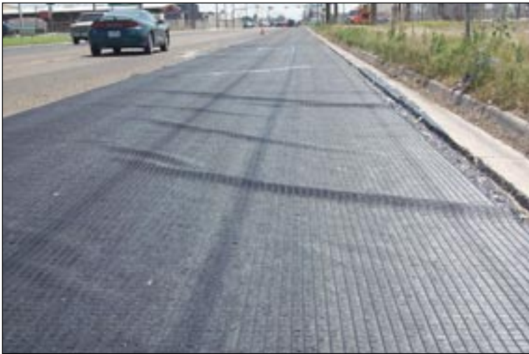
Figure 13. Wrinkles in the geosynthetic surface.
