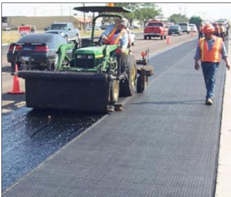
Figure 9. Placing the geosynthetic roll.
