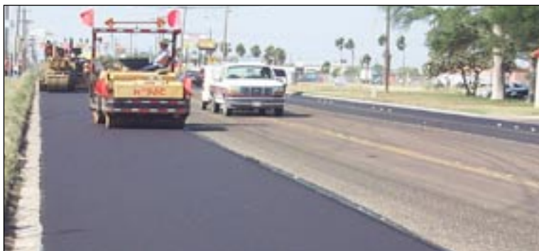
Figure 10. Smoothing the surface.
