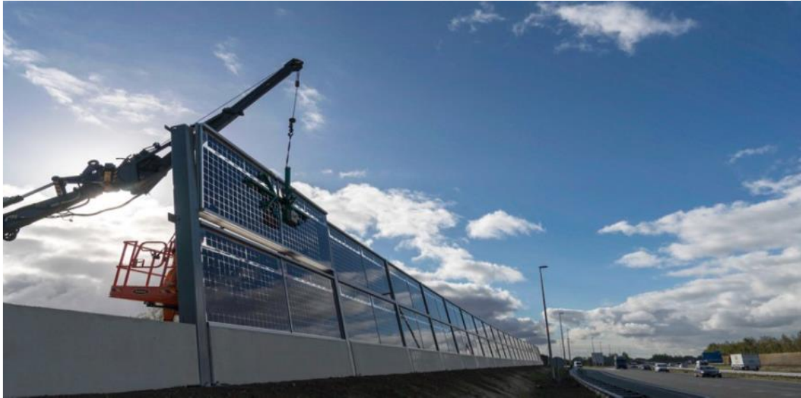
Figure 5. Bifacial PV panels integrated into noise barriers in the Solar Highways project.
