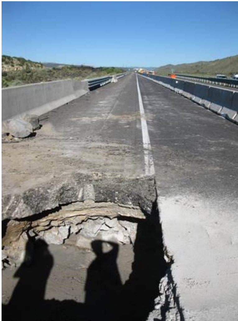
FIGURE 1 Grants, NM Culvert Collapse (Courtesy New Mexico Department of Transportation)
