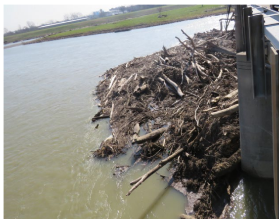
Figure 1. A large debris accumulation at State Route 122 over the Great Miami River in Butler County.
