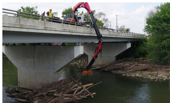
Figure 2. A counterweighted knuckleboom crane with grapple attachment capable of reaching beneath the bridge deck on hammerhead piers.
