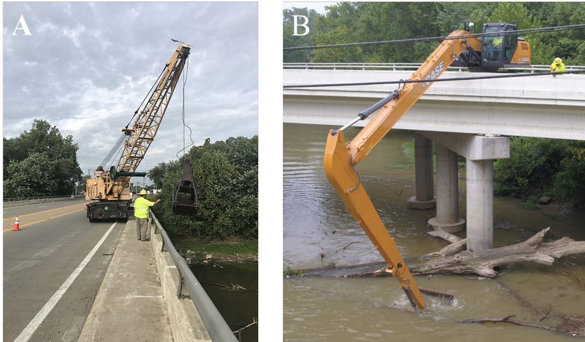
Appendix A Figure 1. A) Lattice boom crane with clamshell bucket, and B) long reach excavator for debris removal.
