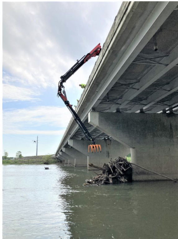
Appendix A Figure 2. Knuckle boom crane reaching below the bridge deck on a tee type pier.
