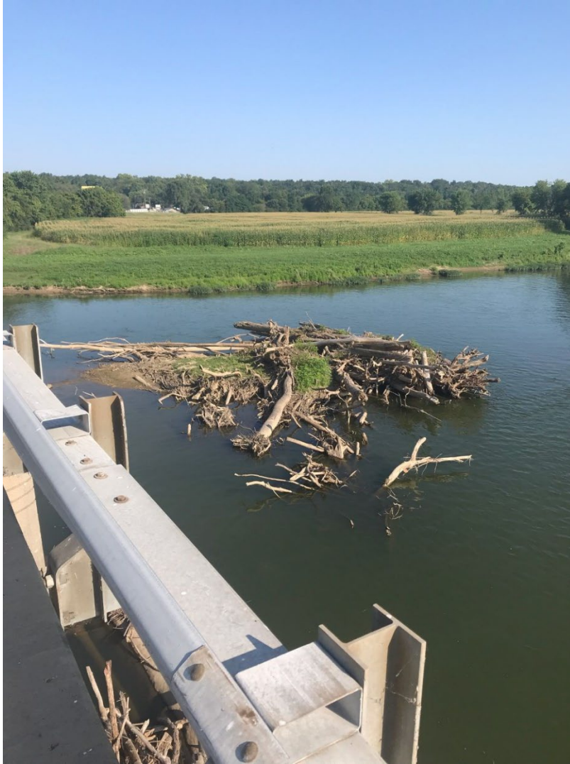
Appendix A Figure 6. Debris accumulation at State Route 122 over the Great Miami River.
