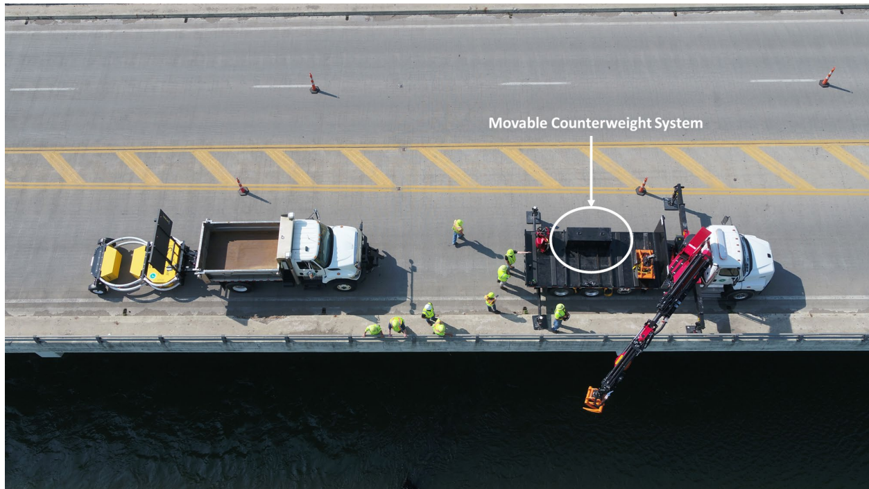
Appendix A Figure 3. Movable counterweight system on knuckle boom truck bed.
