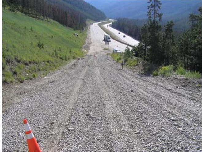
Figure 3.7. Truck Escape Ramp in Colorado (12).
