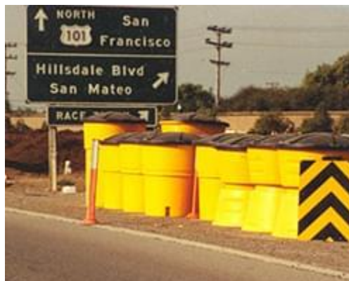
Figure 3.6. Sand Barrel Application (10).
